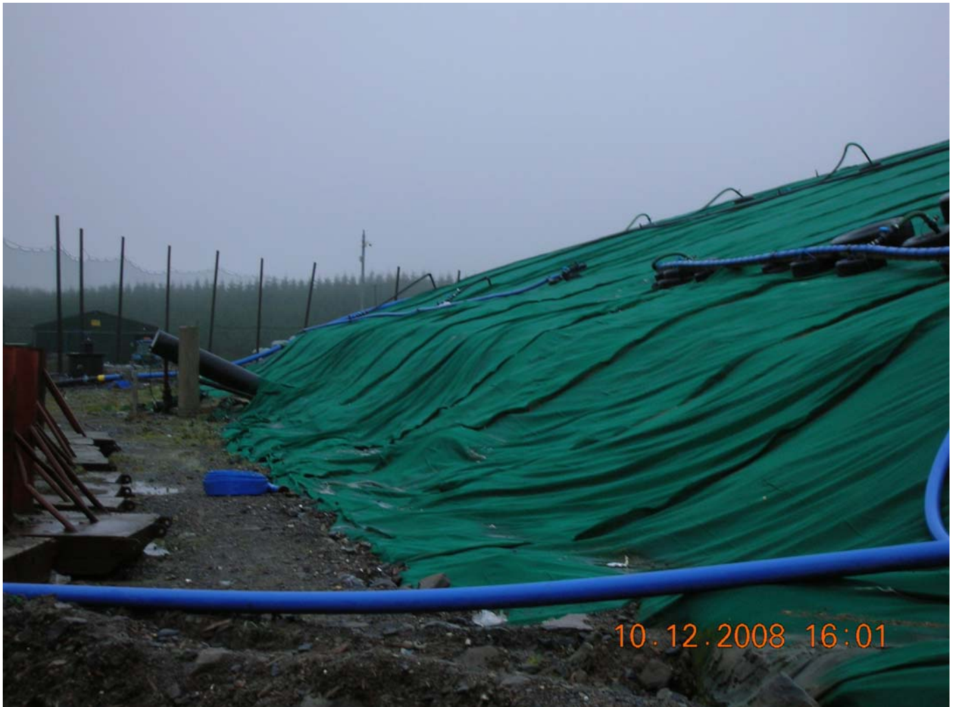
Photo 2: General view of Western Slope
