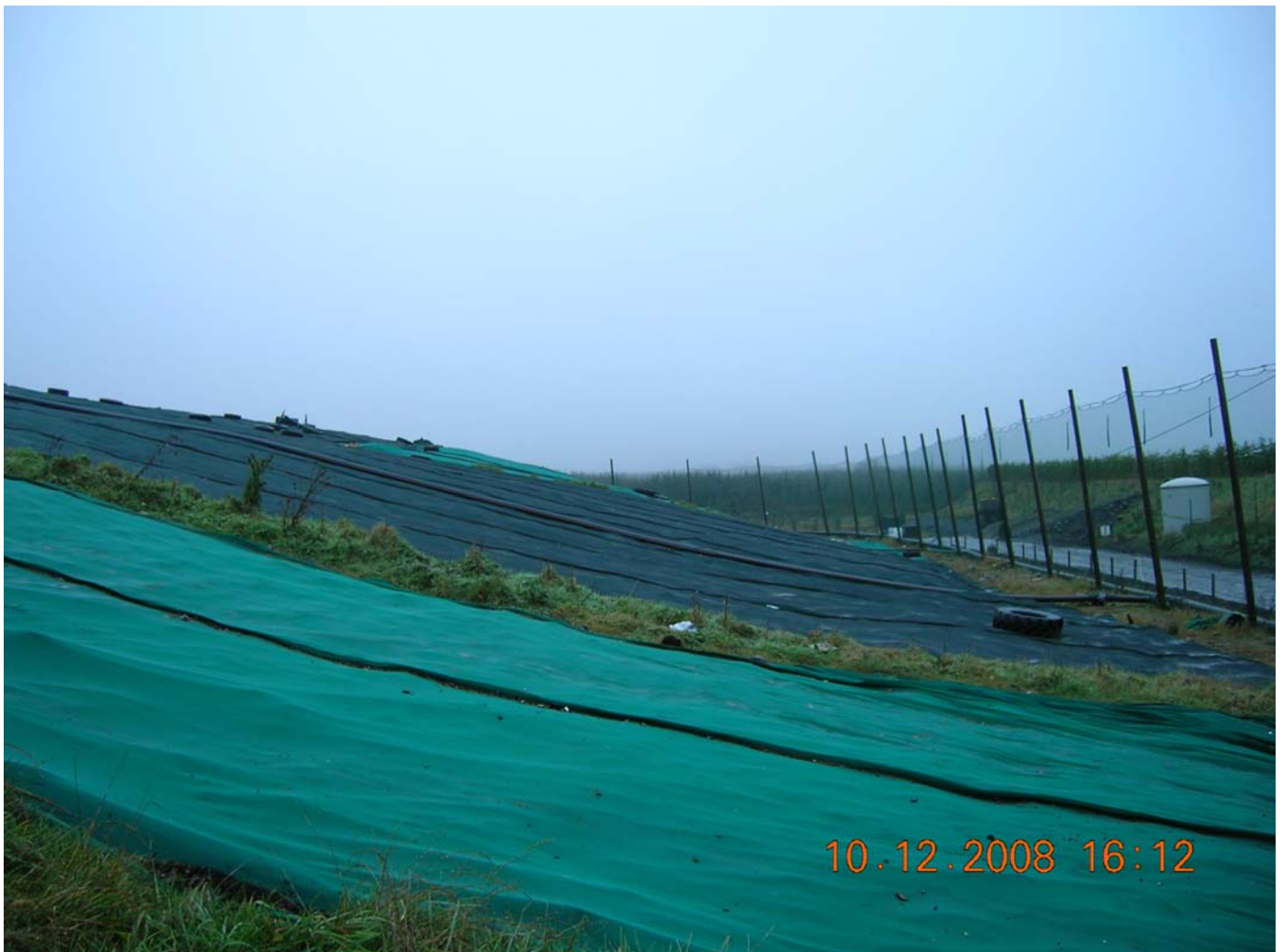
Photo 3: General view of Eastern Slope
