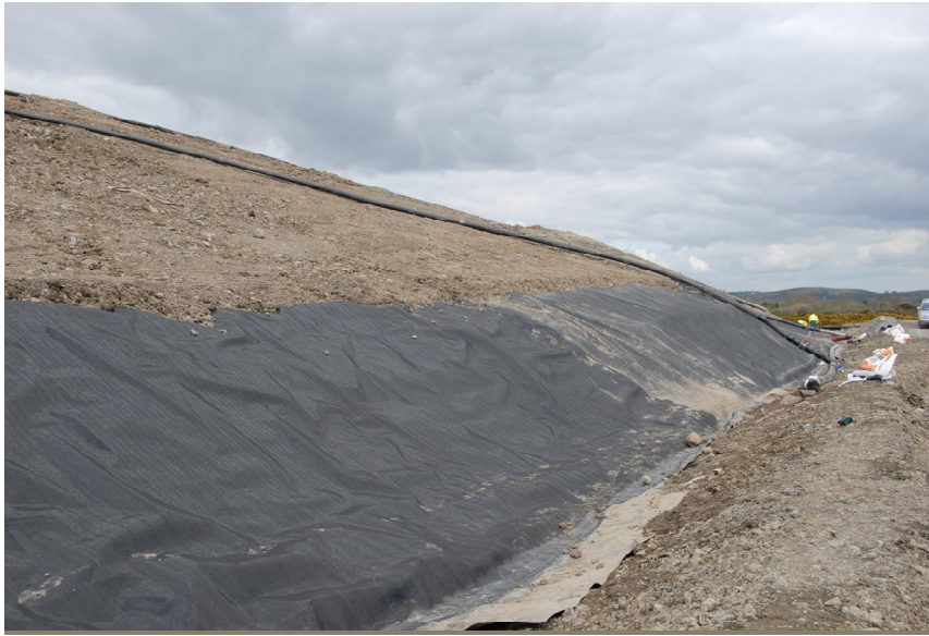
Plate 1: Partial capping material placed on side slopes at rear of Cell 13.
