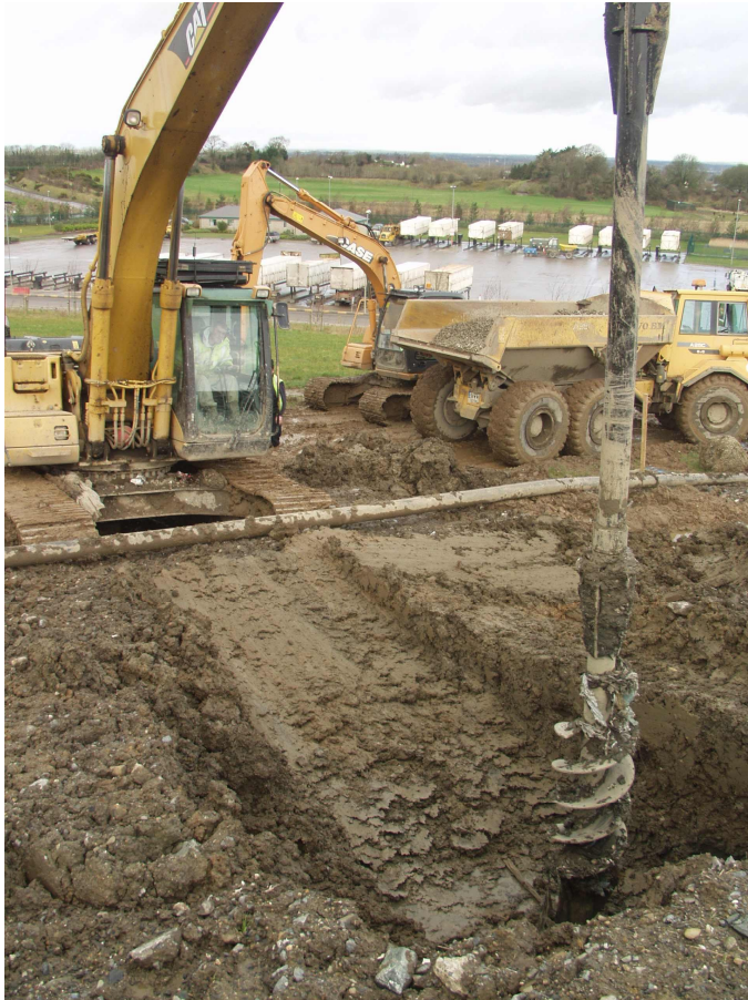
Plate:3 : Auger attached to CAT Excavator. Drilling of new gas wells as deemed necessary by Facility Manager.
