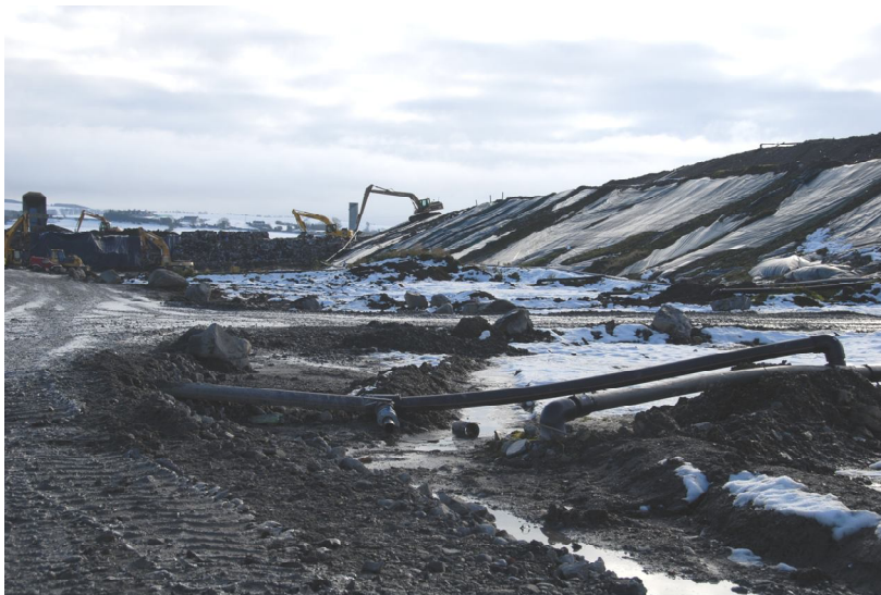
Plate 4: CoverTop 32 placed on side slopes of Cell 14.
