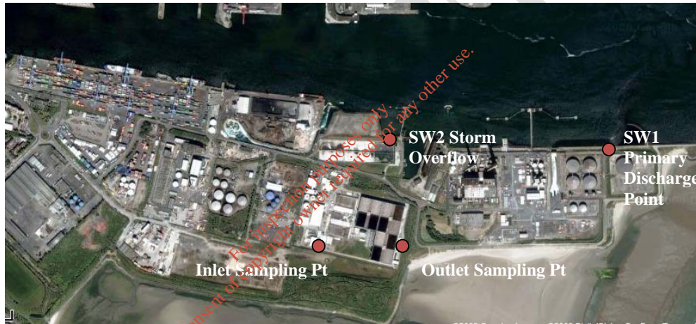
Figure 1: Ringsend Wastewater Treatment Works and Storm Overflow Discharge.
