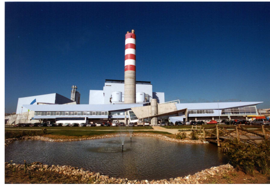
Incinerator in Portugal
