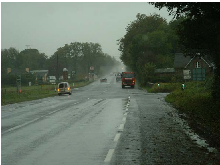
Photograph No 61 N2 / R150 Junction at Flemingstown looking north
