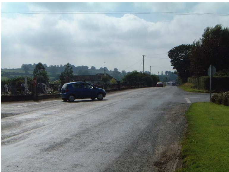
Photograph No 21 R150 Junction at Duleek Looking South (km 10.9)
