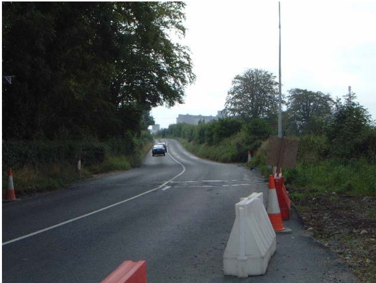
Photograph No 37 Just West of M1 Looking South (km 14.7)
