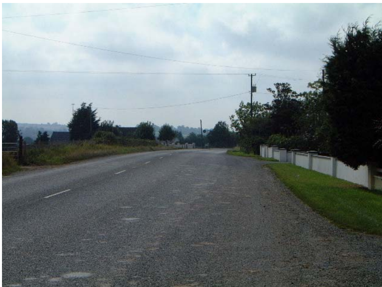
Photograph No 27 Carranstown Looking South (km 12.3)
