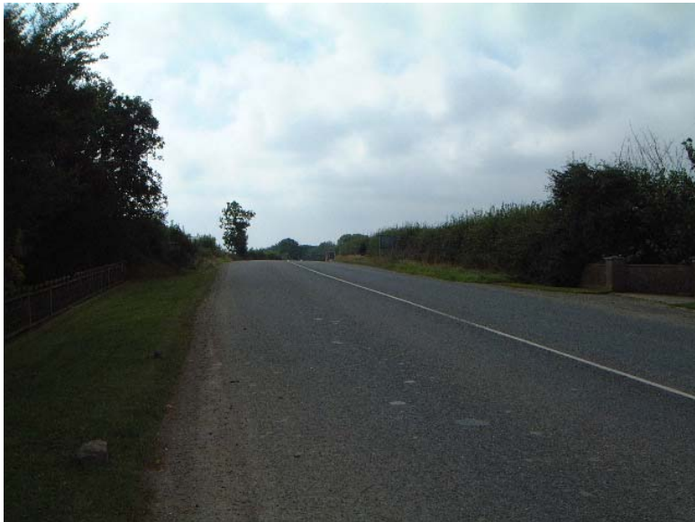
Photograph No 31 Carranstown Kavanagh Centre Looking South (km 13.0)
