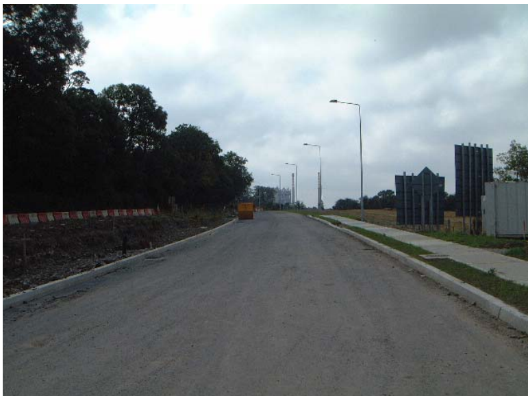
Photograph No 39 Realigned R152 at M1 Junction approach (km 15.0)
