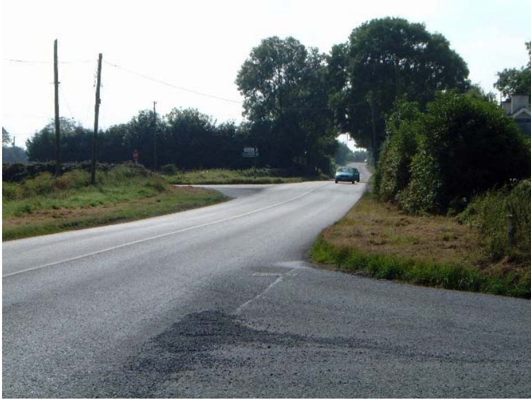
Photograph No 13 Boolies Little Junction Looking South (km 6.7)
