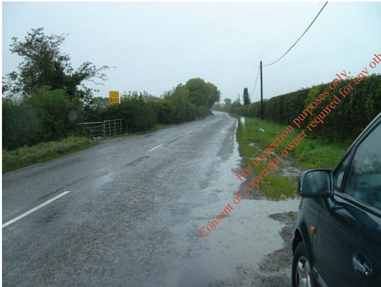
Photograph No 57 R150 looking west at Garballagh, 1.5km west of Duleek
