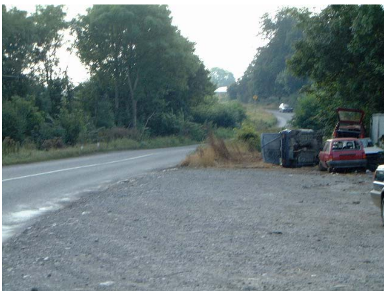
Photograph No 15 Boolies Little Junction Looking South (km 7.0)
