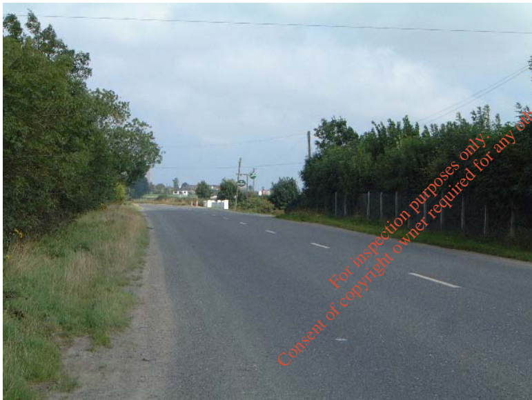
Photograph No 26 Carranstown Inn Looking North (km 12.0)
