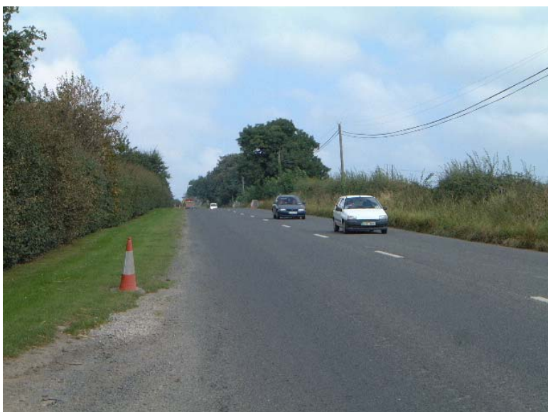
Photograph No 36 Irish Cement Platin Looking North (km 13.9)
