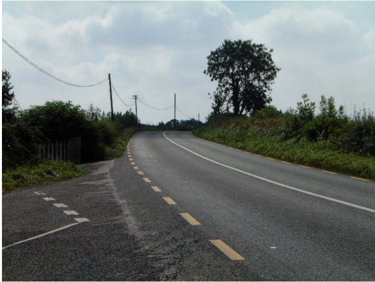
Photograph No 4 Hawkinstown Junction Looking South (km 2.2)
