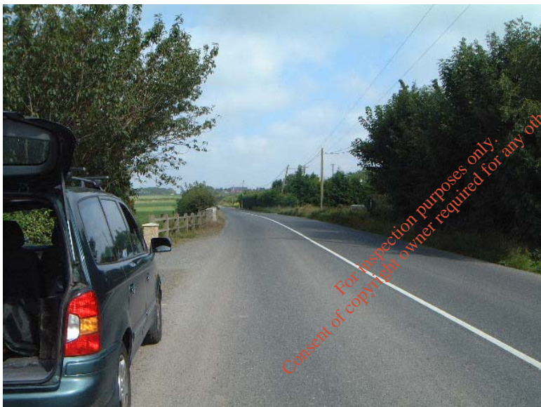
Photograph No 11 Scatternagh Looking North (7.7m wide road)
