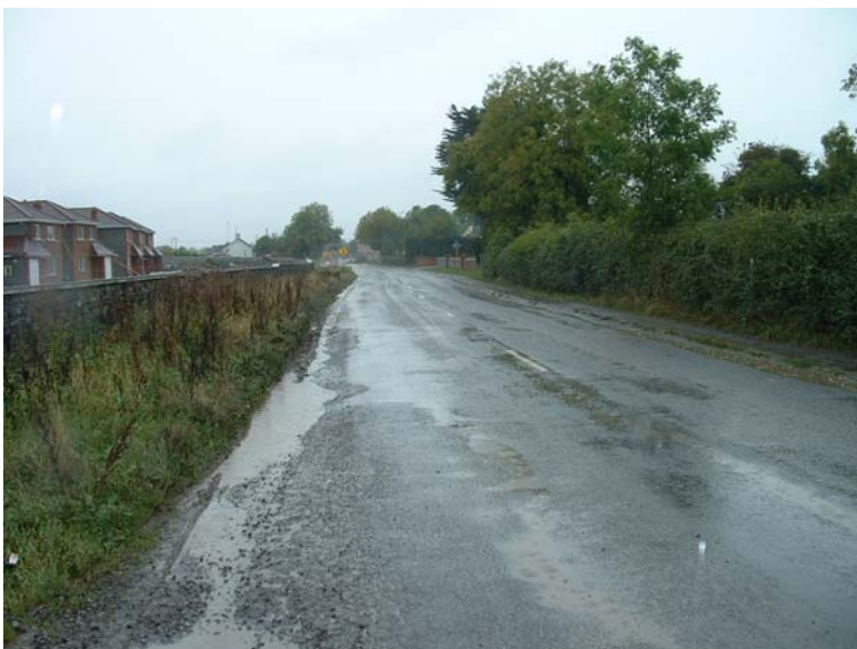
Photograph No 55 R150 at western end of Duleek looking west
