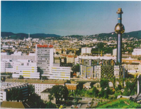
waste to energy facility, Vienna City Centre
