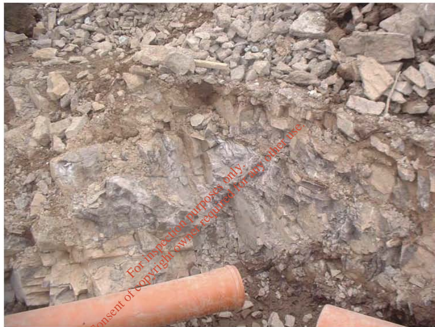
Plate 1: Weathered Bedrock exposed along site excavations
