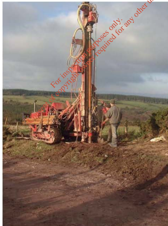
Plate 2: Drilling of Groundwater Monitoring Boreholes
