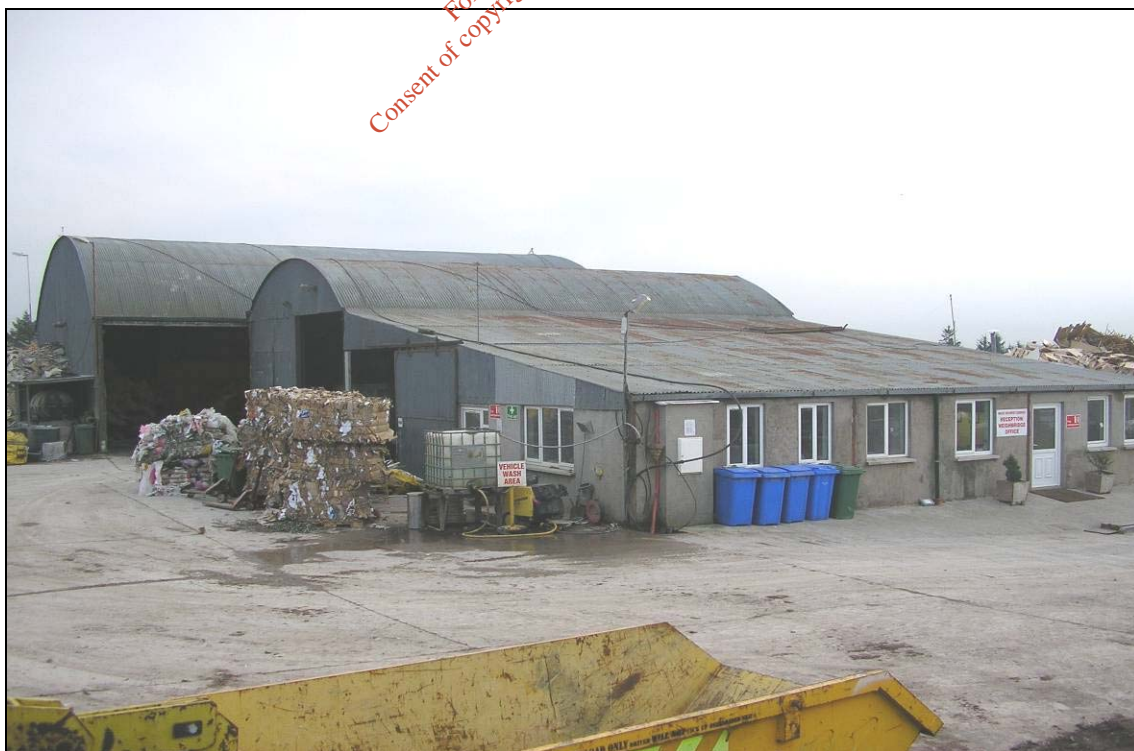
Plate 2. Main site buildings.
