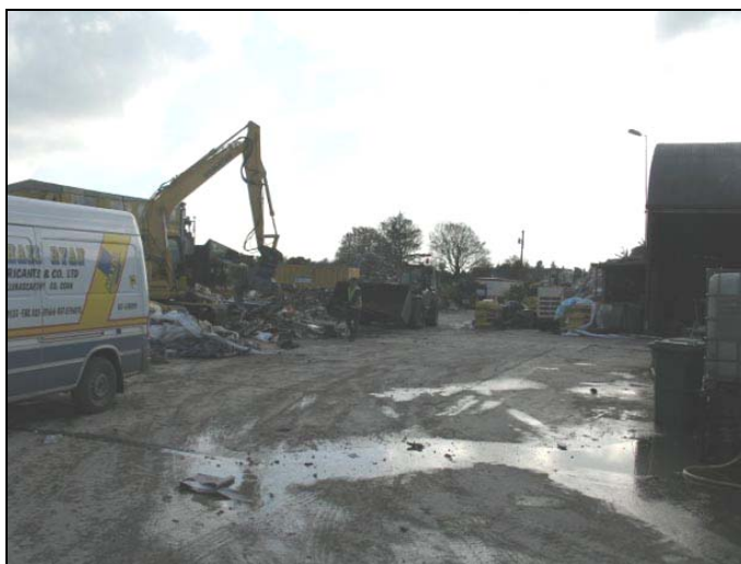
Plate 1. View of proposed site of new building from north.
