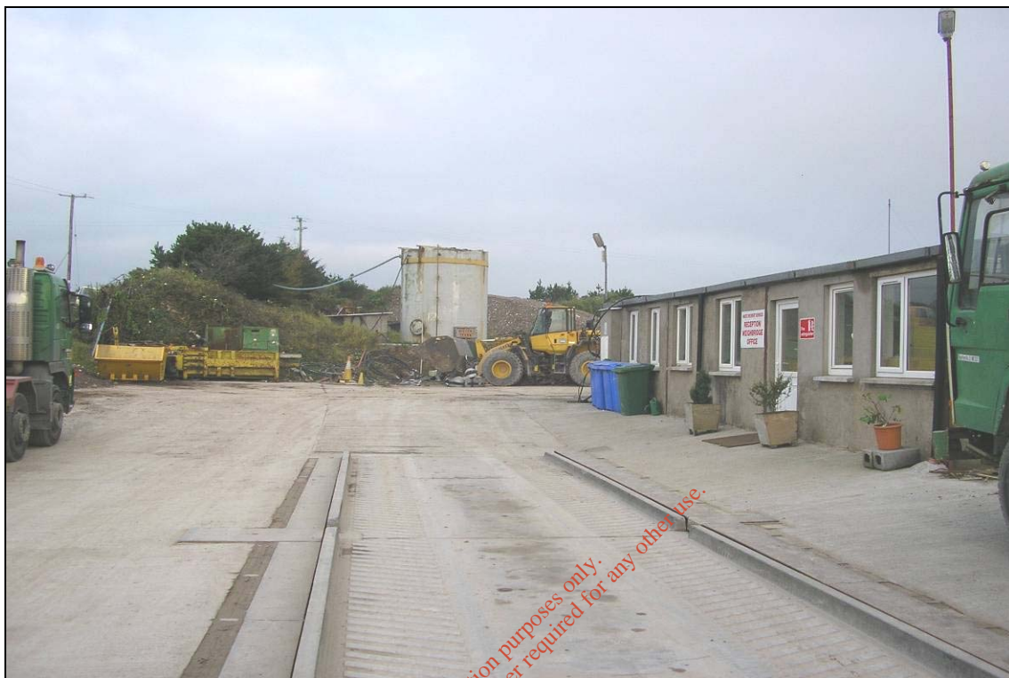
Plate 1. Weighbridge and offices.
