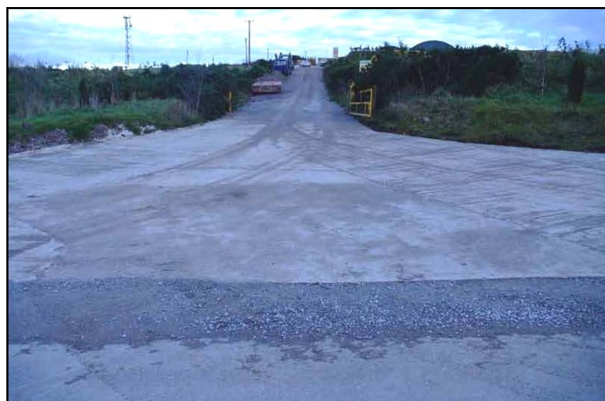
Photograph 3. View into Site Access from County Roadway.
