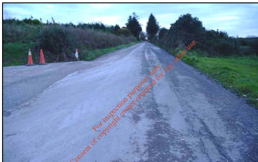
Photograph 2. View Along County Roadway to South.
