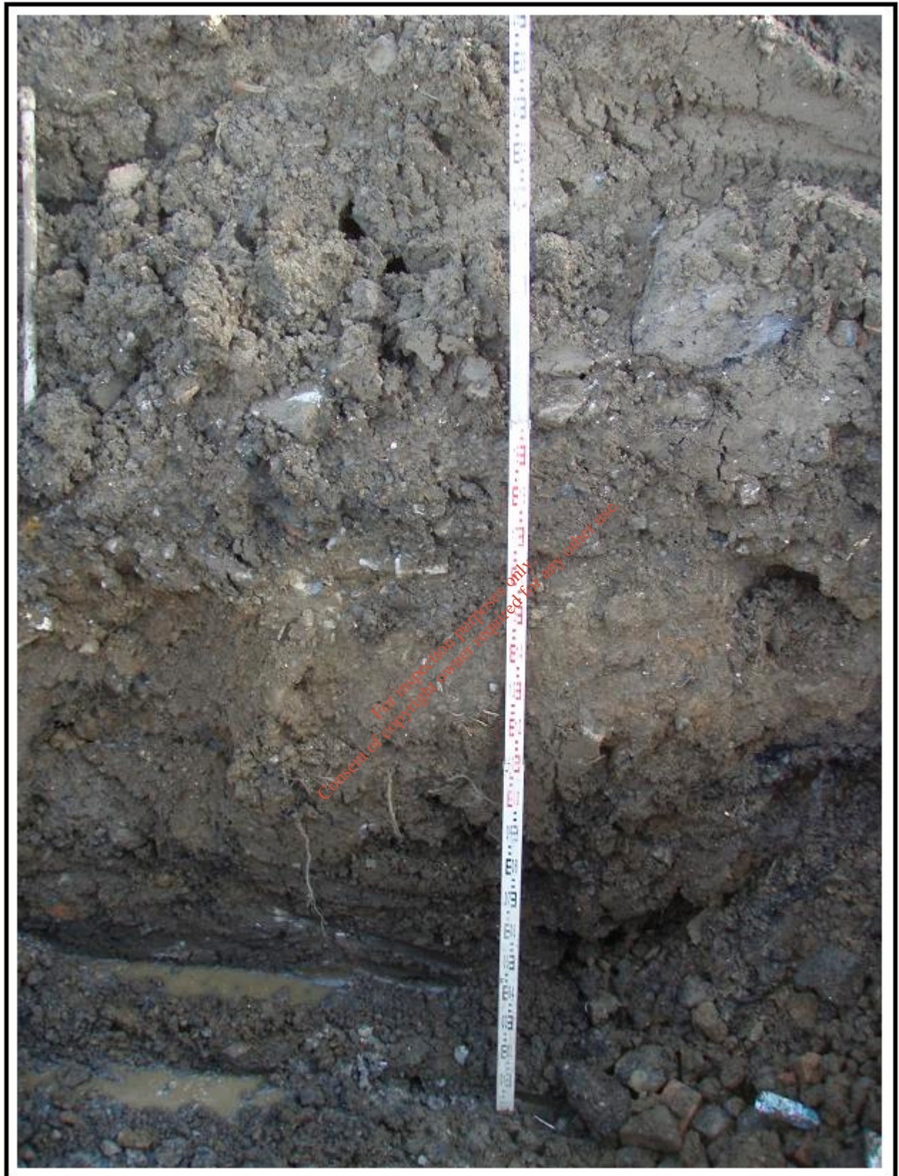
Plate A8: Profile of recently-filled subsoil in trial hole no. 8. Pieces of concrete, bricks, wire, branches and plastic piping are seen occasionally, within alternating layers of compacted subsoil.
