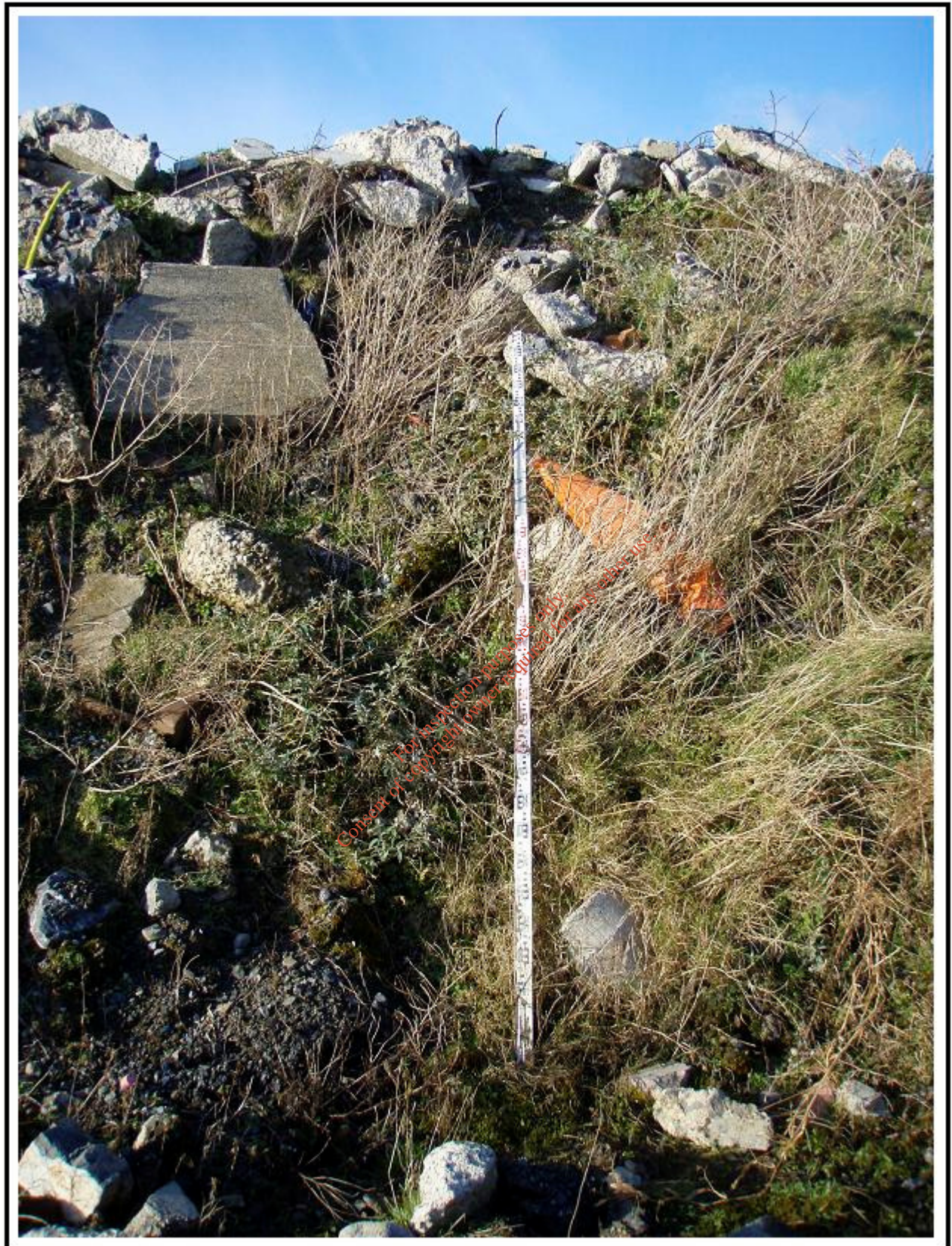
Plate A14: Profile of recently-lain consolidated subsoil at the eastern edge of the main (western) fill area. Though containing much construction and demolition material at the face, this material is also relatively clean throughout.
