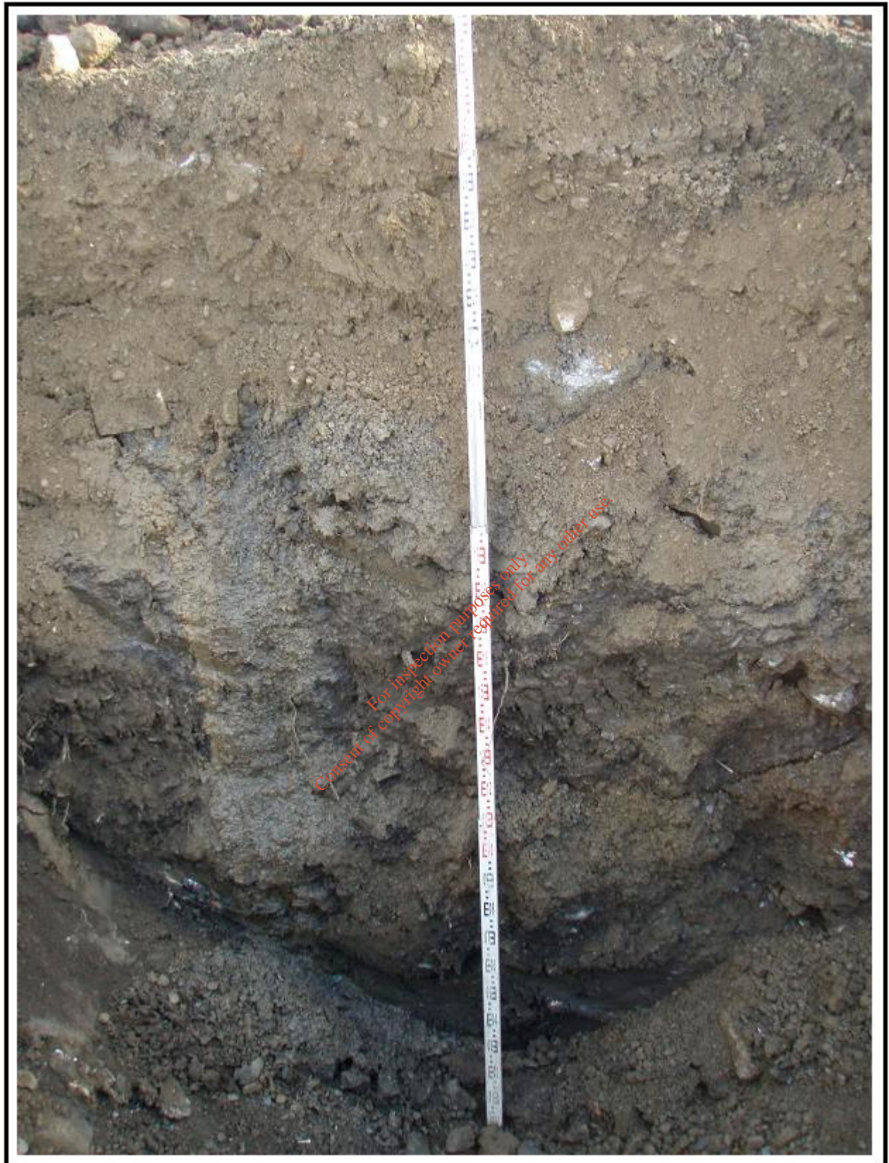
Plate A6: Profile of recently-filled subsoil in trial hole no. 6. Pieces of concrete and boulders are common in this area of the site also, with alternating compacted layers and occasional construction and demolition material.
