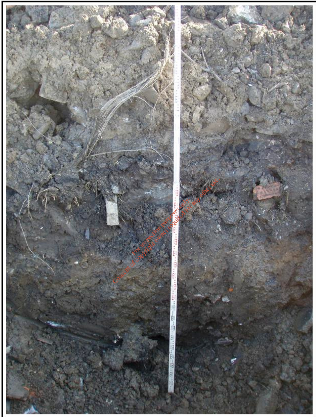
Plate A7: Profile of recently-filled topsoil and subsoil in trial hole no. 7. Pieces of concrete, bricks, steel, wire and plastic are seen occasionally, within alternating layers of compacted subsoil.
