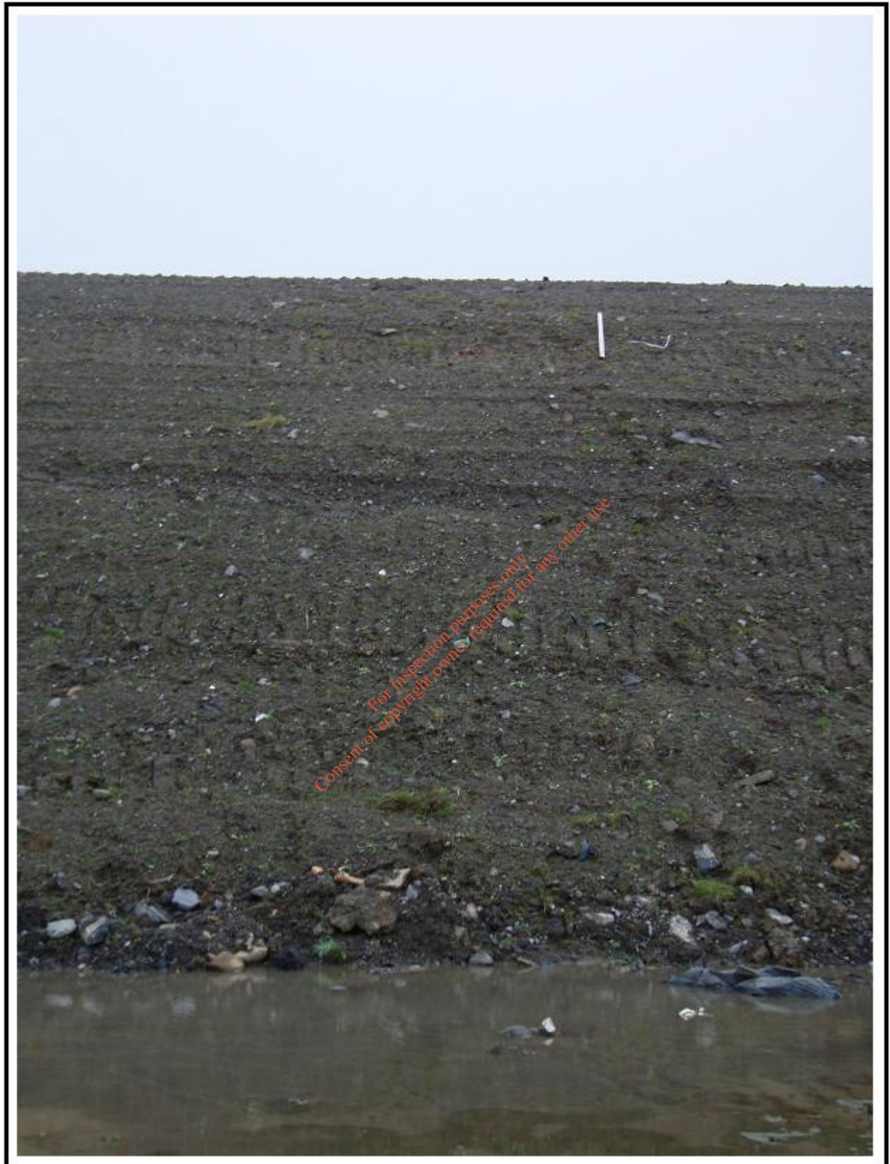
Plate A15: Profile of relatively shallow, recently-lain topsoil overlying overconsolidated subsoil at the northern side of the main eastern fill area. This material is very clean also.
