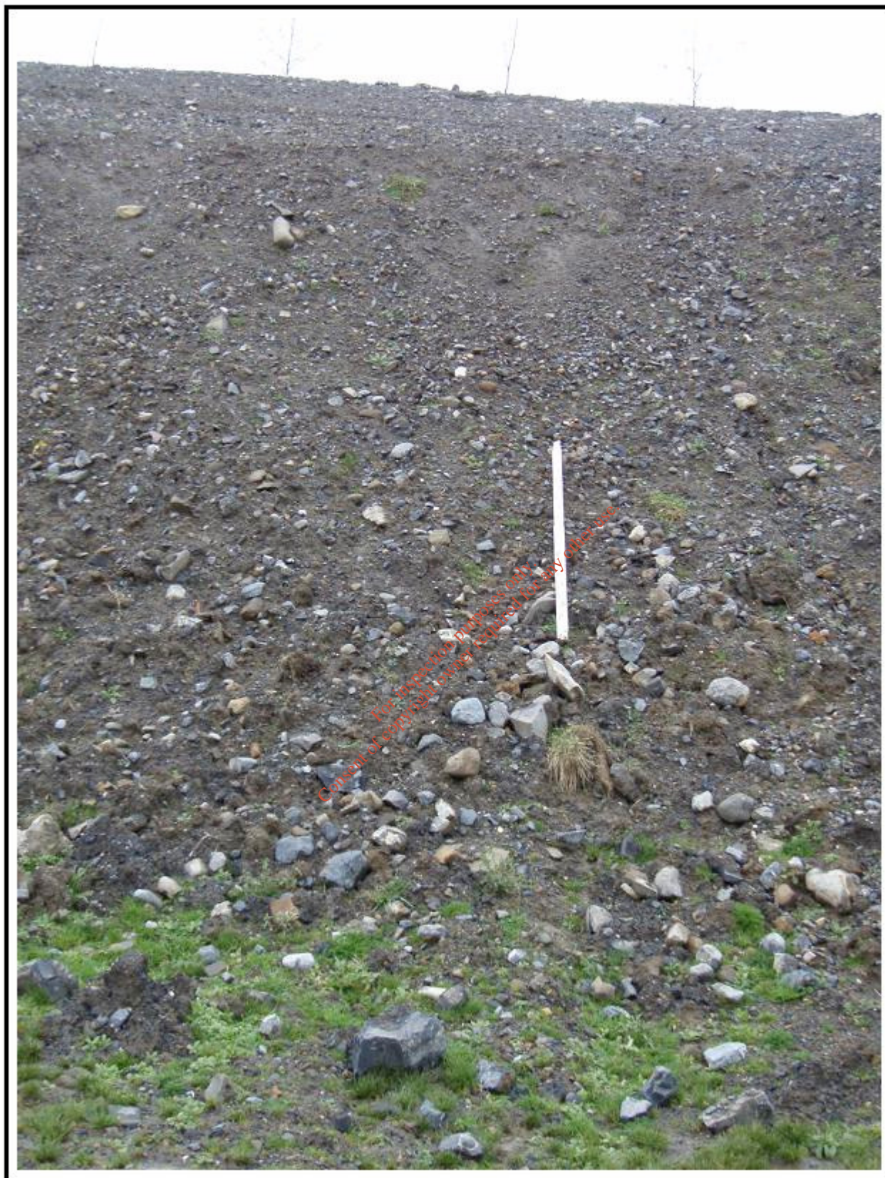
Plate A18: Profile of exposure into subsoil at the northwestern extreme of the main pit area. This material is clean, and again gets more gravelly and 'bouldery' at the base.
