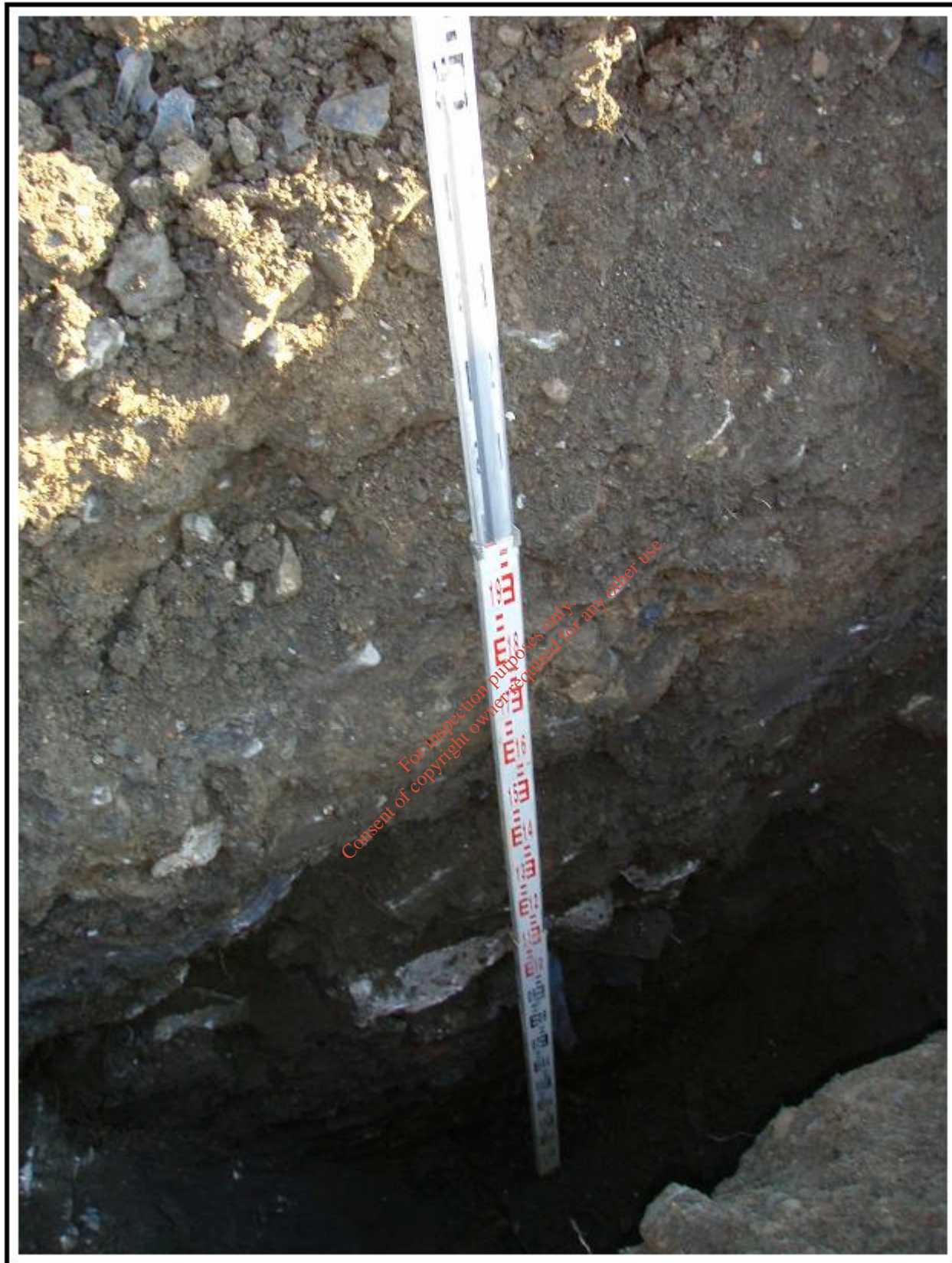
Plate A11: Profile of overconsolidated subsoil with alternating layers of very soft to stiff material in trial hole no. 11. Here some buried pieces of concrete are seen at depth. No topsoil has been emplaced above this material as of yet, and the ground is bare.
