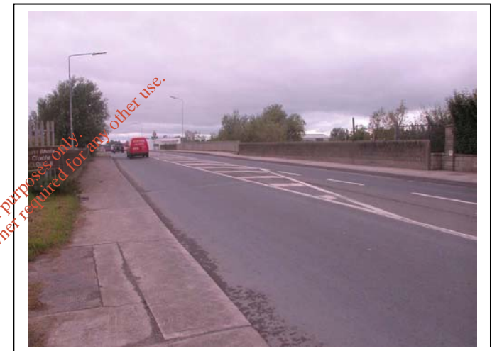
Plate 11.21: Location of Bawney Bridge, Dock Road from east
