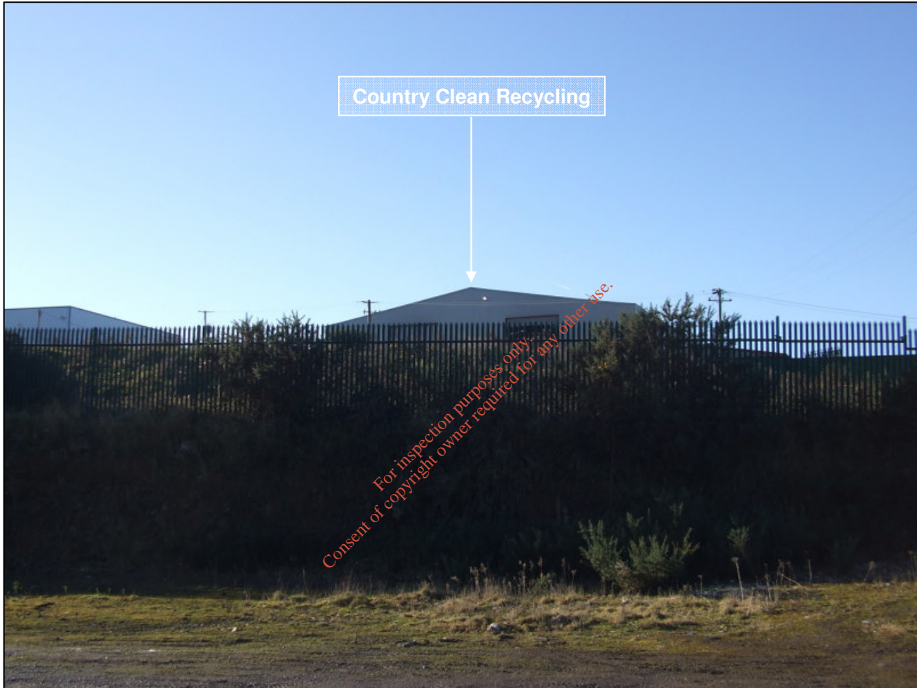
View 9: View from Ard Alainn, off Upper Fairhill road looking southwest towards Country Clean Recycling Ltd.
