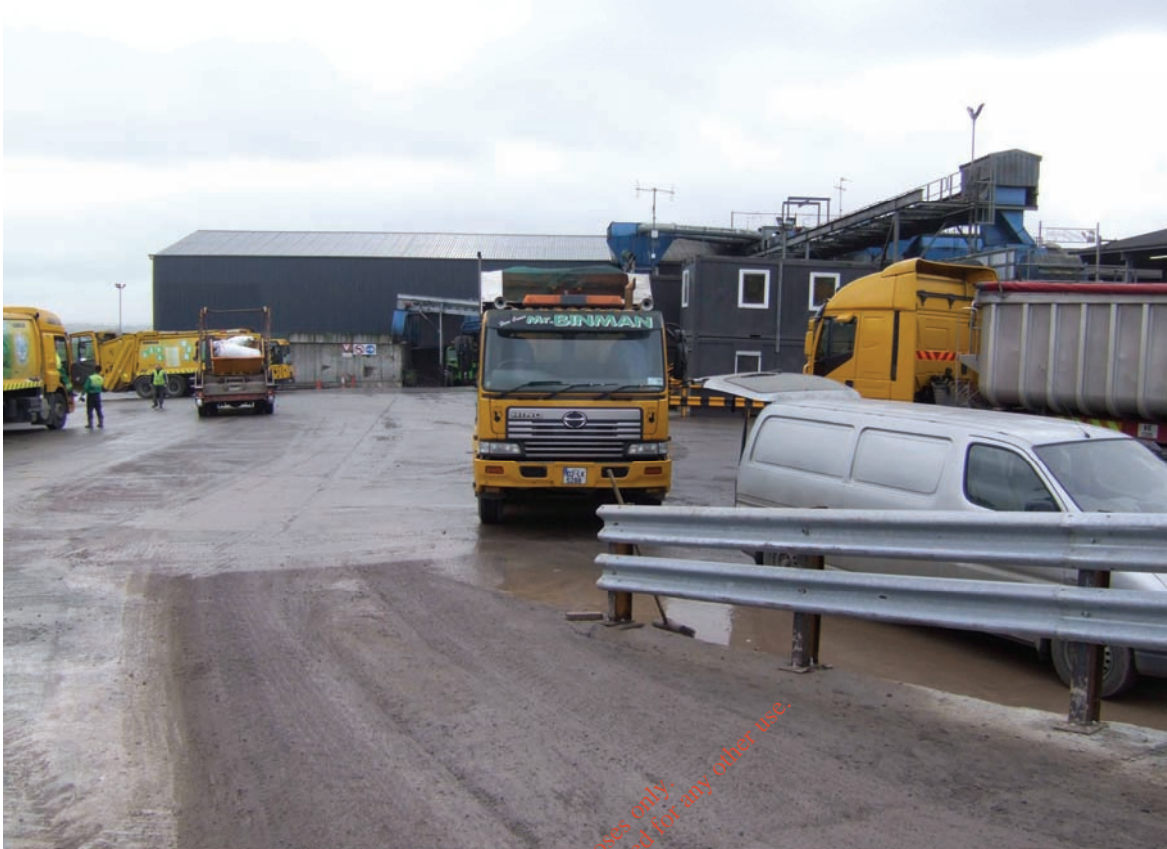
Plate 5.1. Showing some of the buildings and hard standing on the site.
