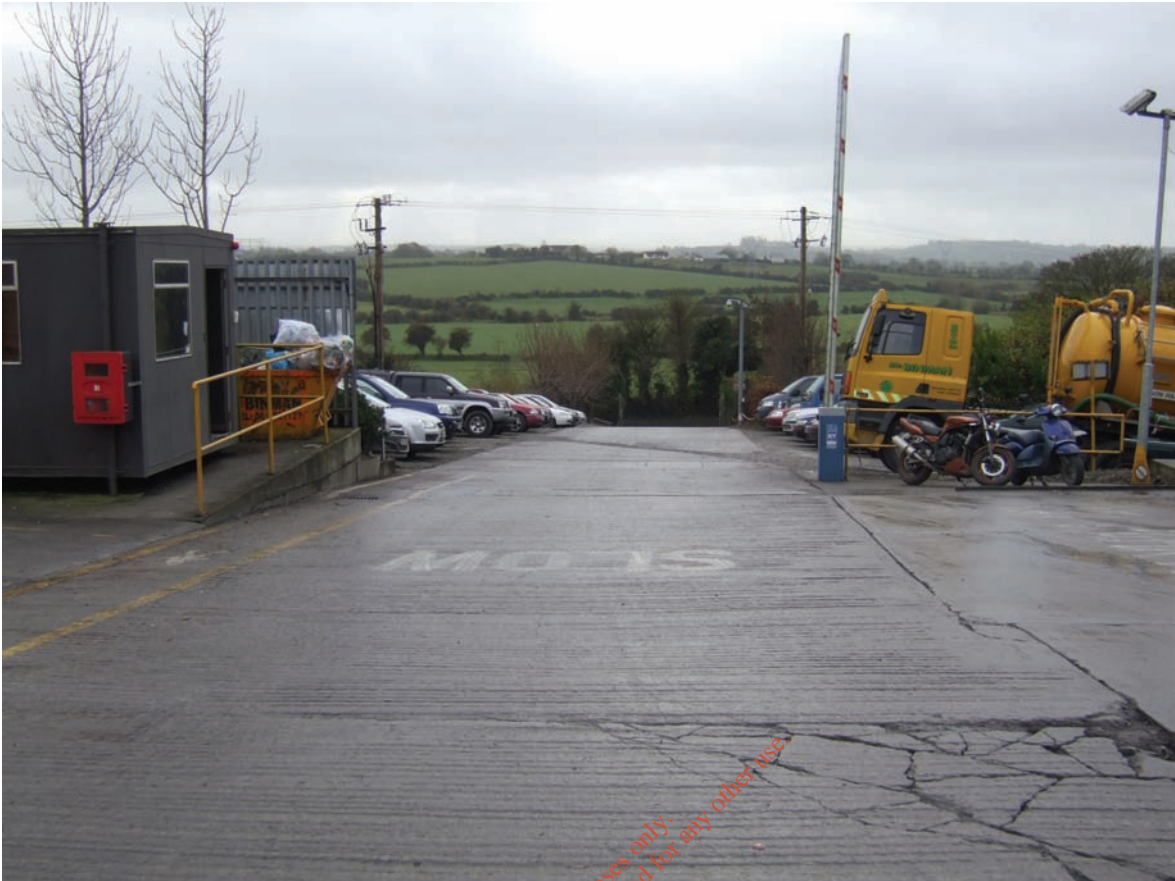
Plate 3.15 Entrance roadway utilised by waste collection trucks
