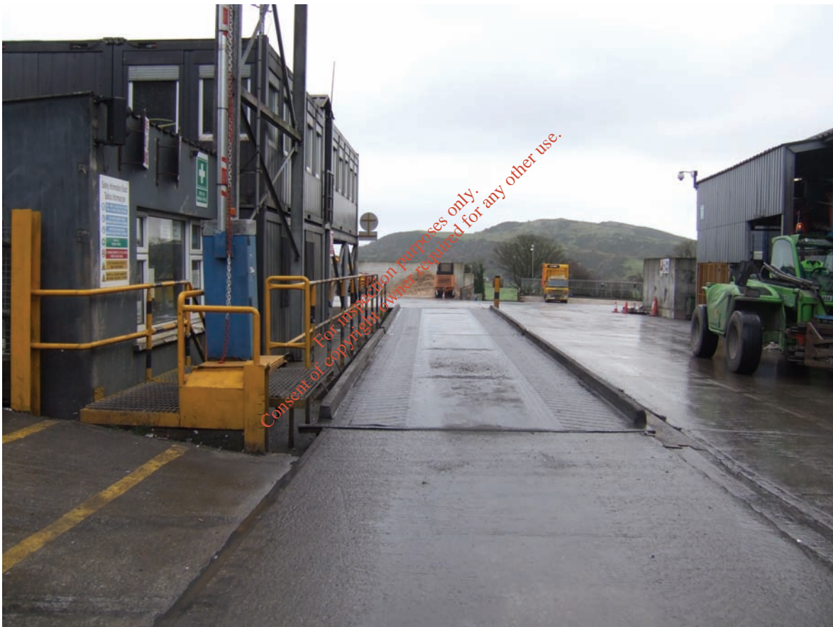
Plate 3.1 Weighbridge at the waste transfer station
