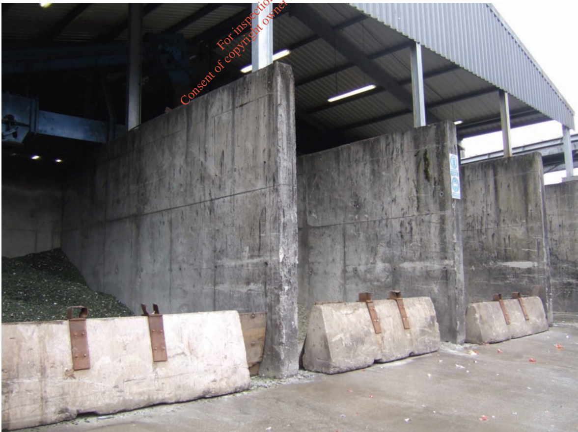
Plate 3.5 Storage bunkers for crushed glass
