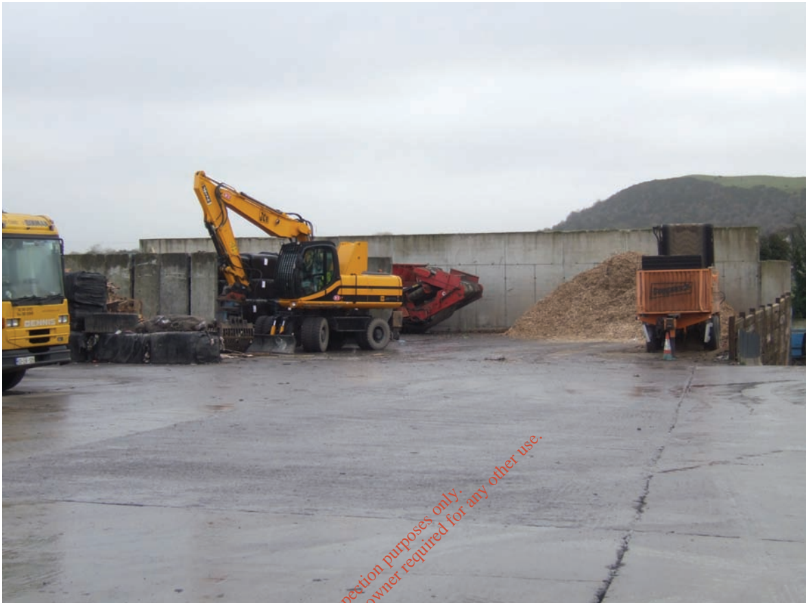
Plate 3.7 Timber Processing Area
