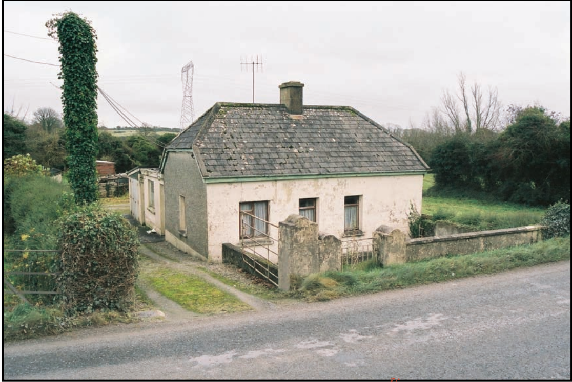
Plate 10.5 SITE CH-4 (from northeast)
