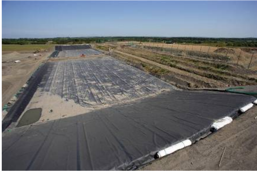
Plate 3.2 Lined cells at Knockharley Landfill
