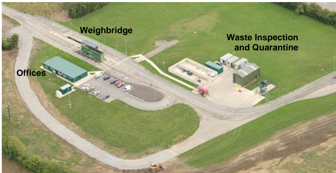
Plate 3.1 Knockharley Landfill Administration Buildings
