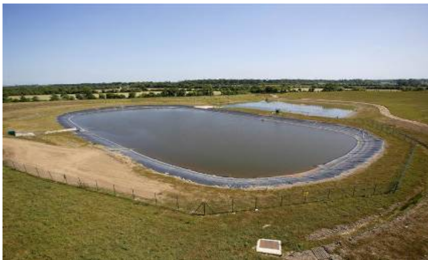
Plate 3.3 Storm Water Attenuation Pond
