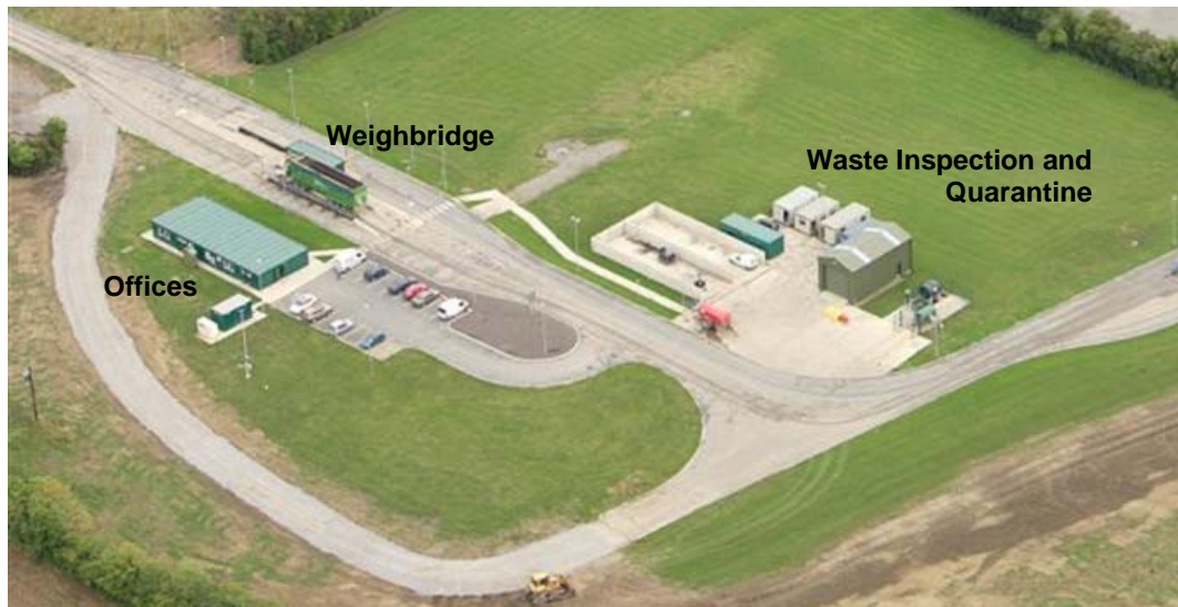
Photograph 1.1 Knockharley Landfill Administration Buildings
