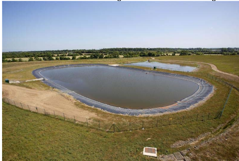
Photograph 1.3 Storm Water Attenuation Pond
