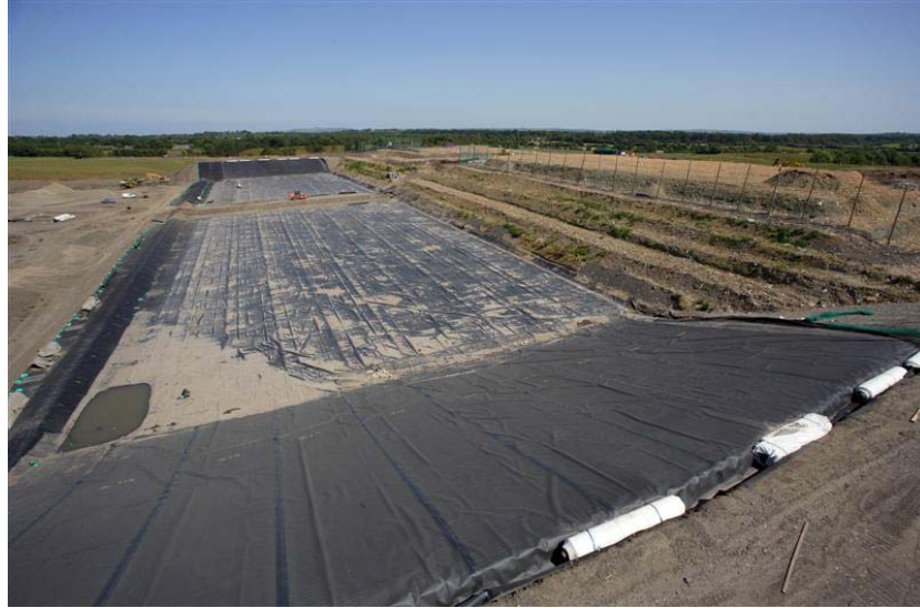
Photograph 1.2 Lined cells at Knockharley Landfill
