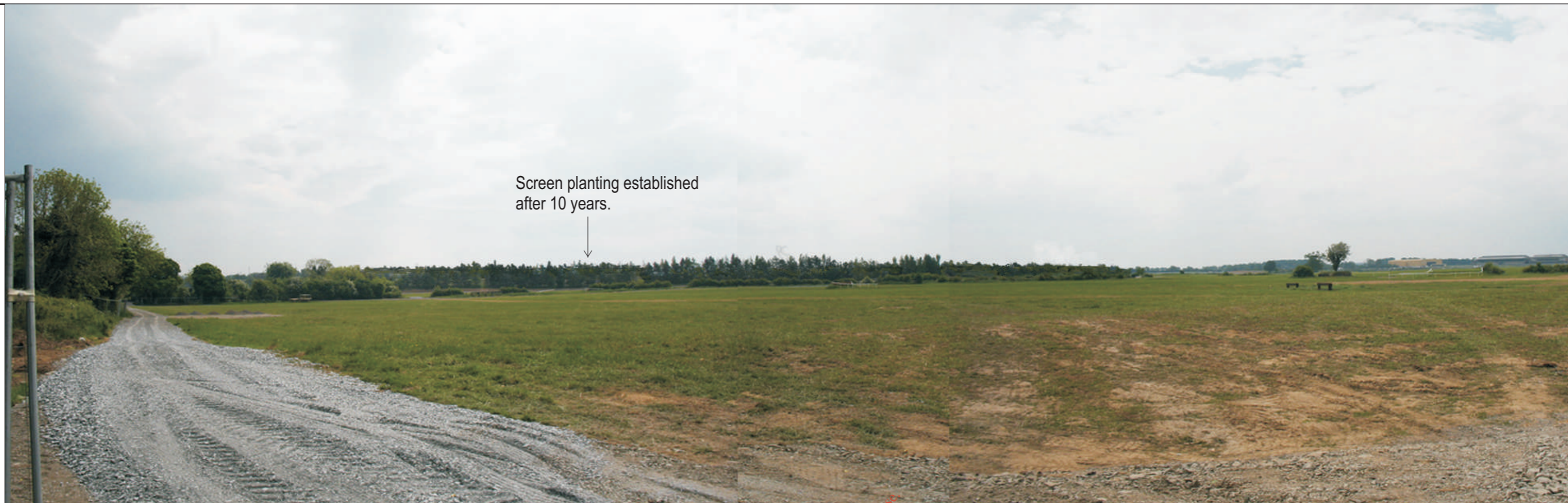
Photomontage viewpoint 1: Across from the L6042 road to the north of the site looking across Punchestown Racecourse - View during Operational Period (10 years)
