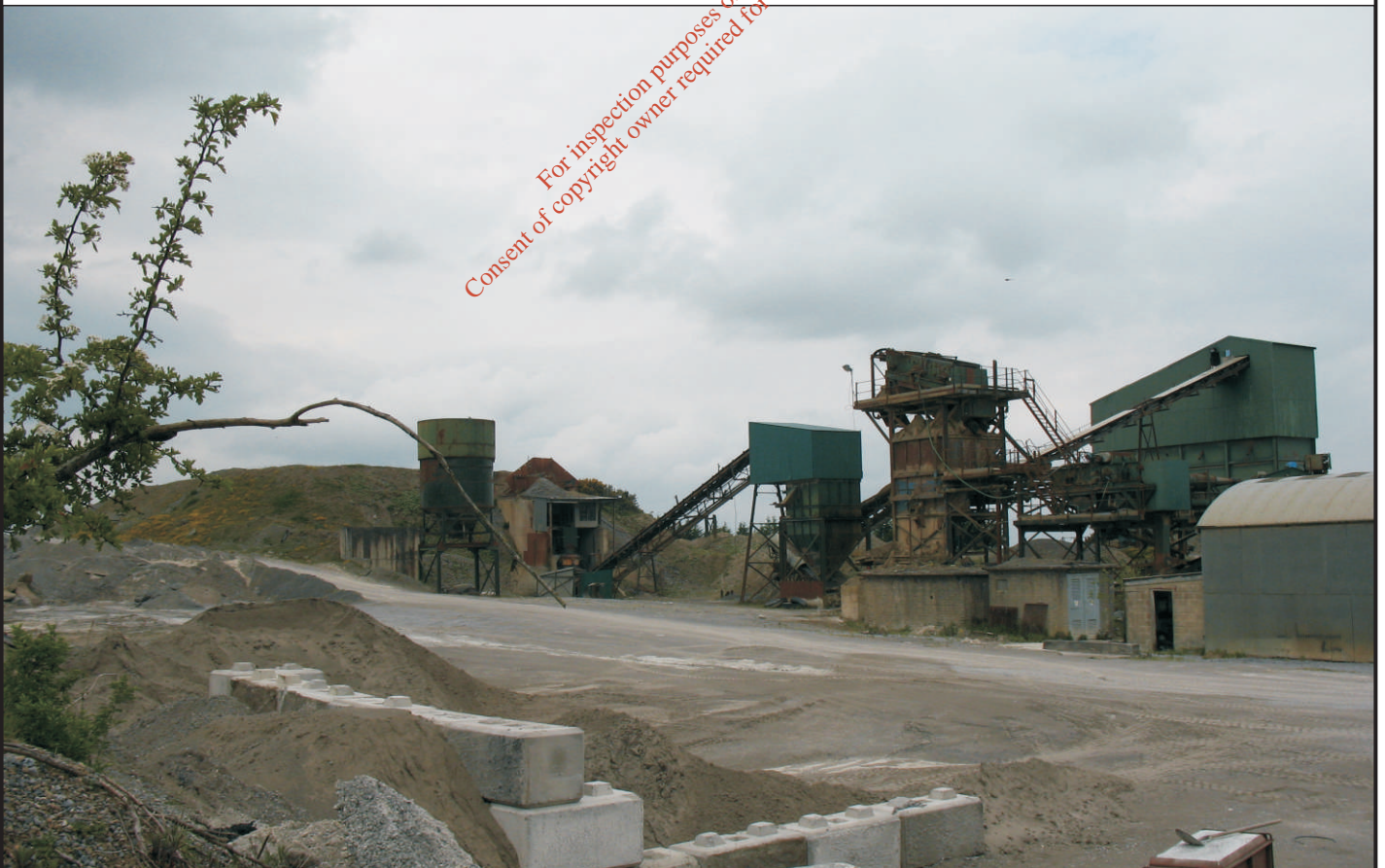
B- View of concrete batching plant and redundant processing plant
