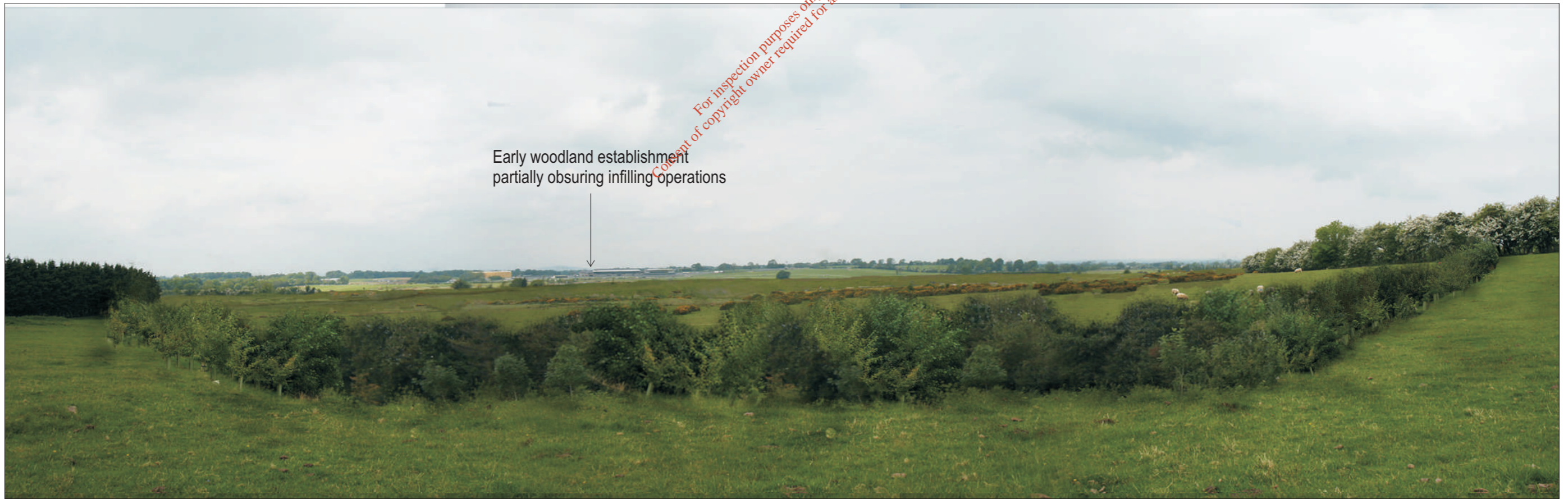
Photomontage viewpoint 2: Across from residential property to the east- During Early Site Establishment (after 3 years)
