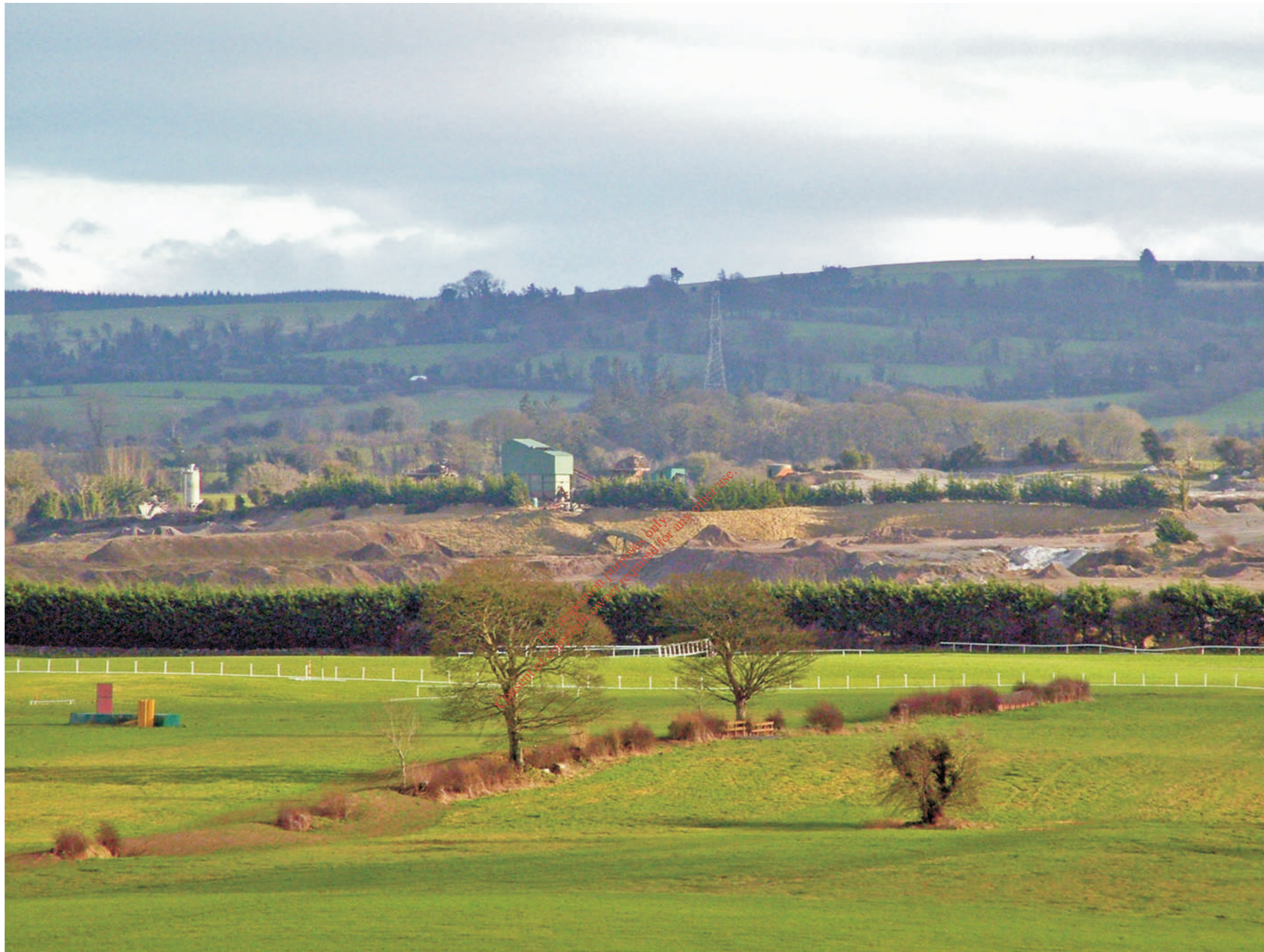
16.3 (a) Existing view looking east towards Cemex lands from Punchestown Stand.
