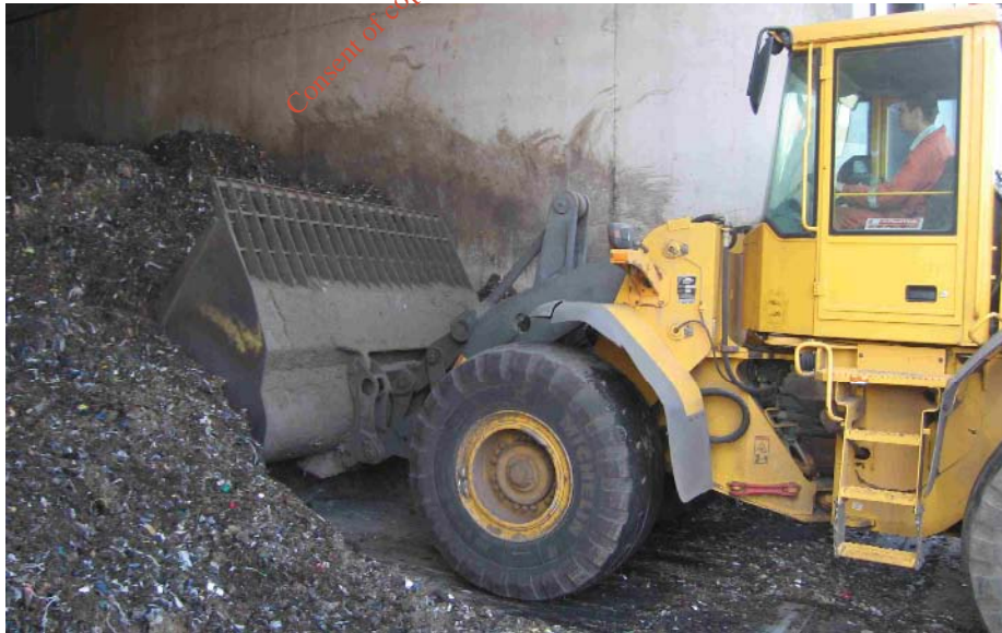
Front-end loader removing material from concrete tunnel
