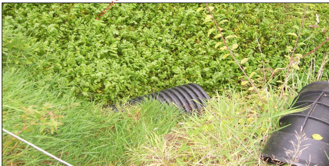
Plate 3.2.6 South Drainage Ditch looking east
