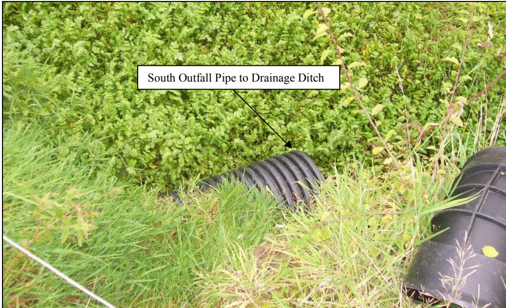
Plate 3.4.1 South Drainage Ditch looking east
