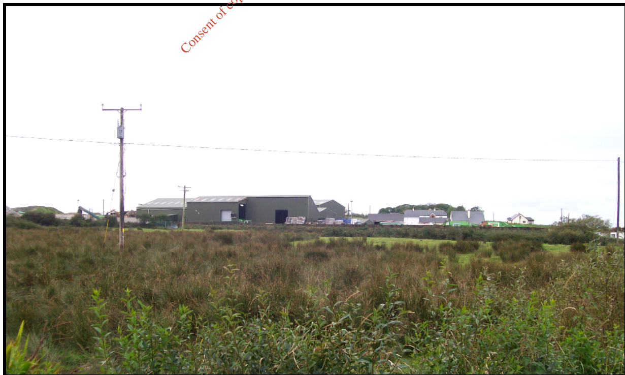
Plate 2.4 View of east face looking west
