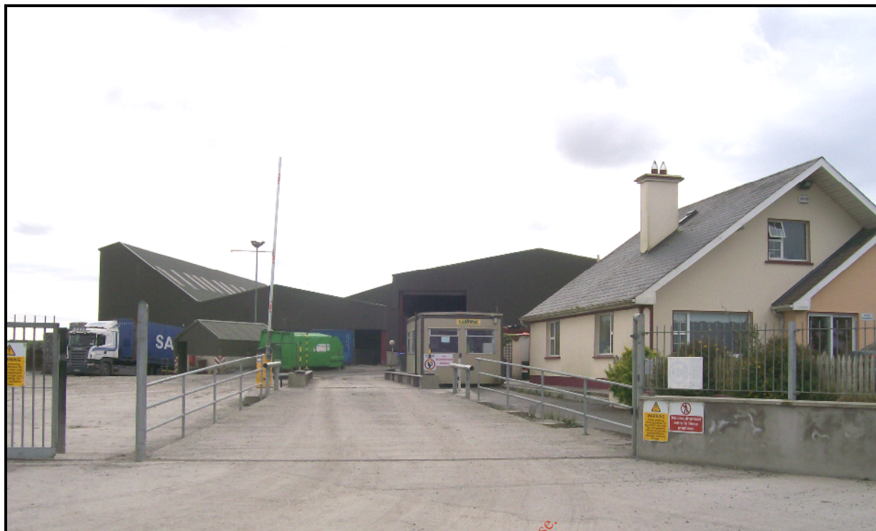
Plate 2.2 Front of facility looking south
