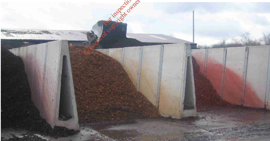
Outdoor product storage bunkers
