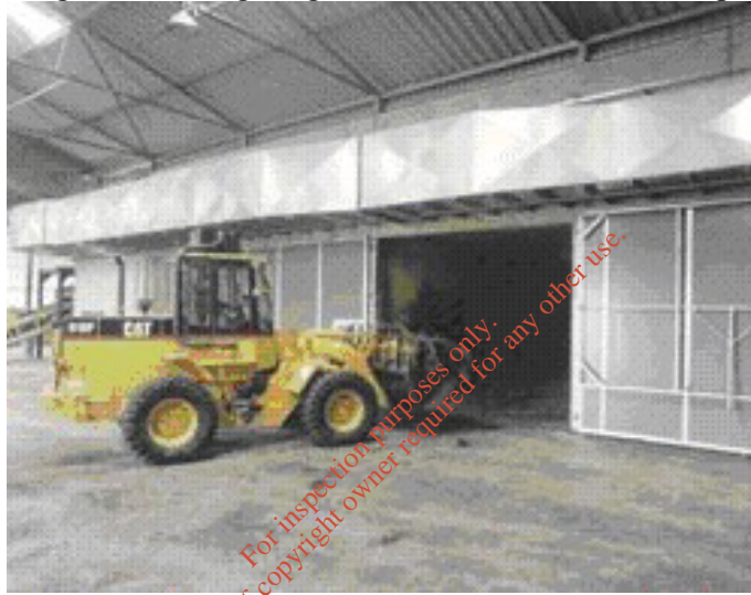
Loading a fully enclosed composting tunnel with a front-end loader
