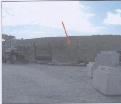
Plate 7: Existing berm at W side of site, looking W.
