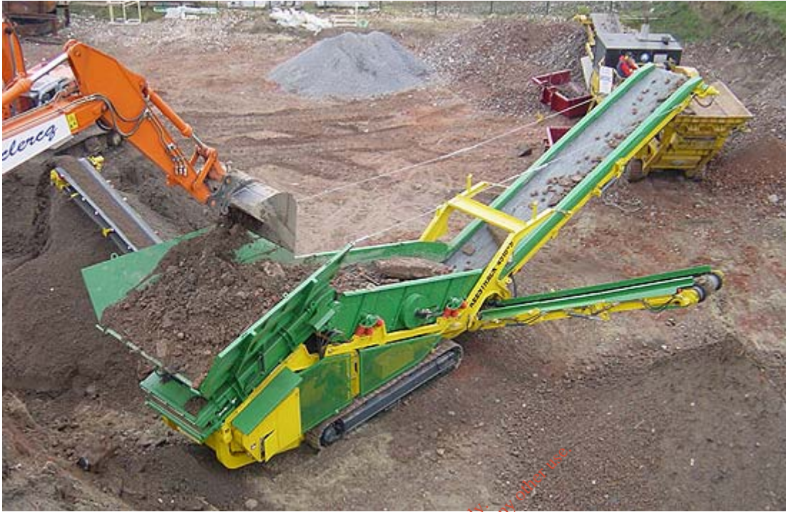
Figure D2.2 Shows Pioneer Equipment to be used on site
