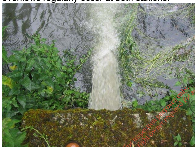
Figure SW05Dway-02 - Overflow from Quarry Road Pumping Station
