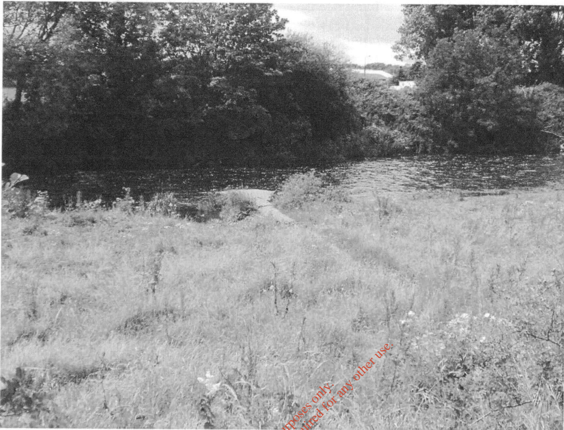
Photograph C2-1: SW03-Kant, Overflow from pumping station
