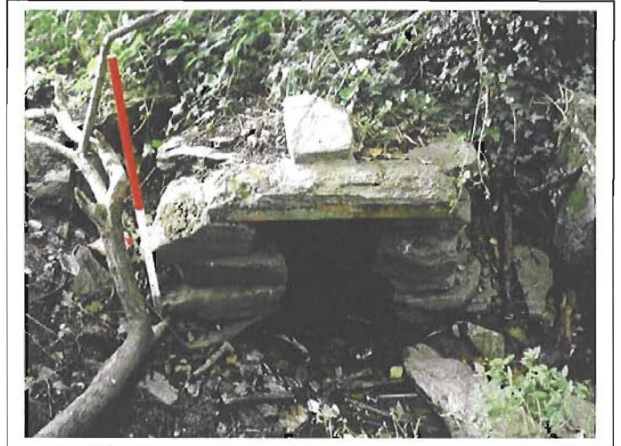
Plate 3.36. CH2, from east
