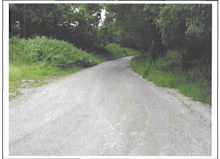
Plate 3.6. Pipe route within ZAP of CH4, in Ballyfouloo, from northeast
