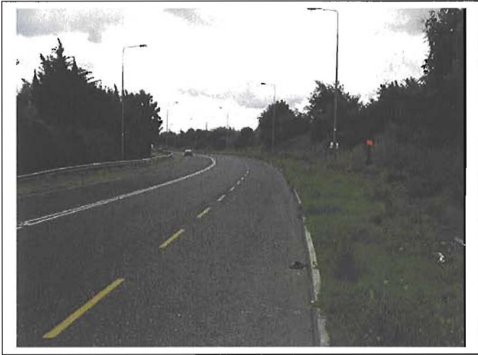
Plate 3.24. Pipe route along N28, from northwest
