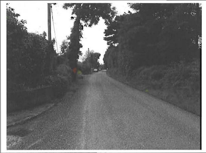
Plate 3.5. Route of pipe along road within ZAP of CH3 in Parkgarriff, from northeast
