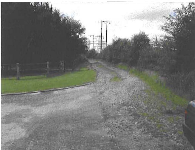
Plate A3 Artificial surfaces - the roadway leading into the proposed wastewater treatment plant site.
