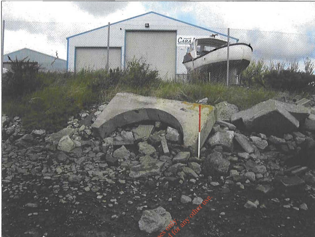
Plate 17: North-facing view of upper foreshore c.100m along pipeline route (see Figure 6 for location); 1m scale.
