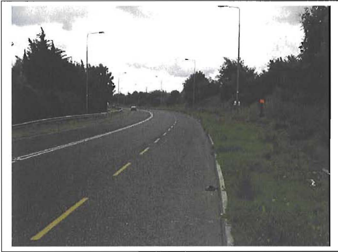
Plate 3.24. Pipe route along N28, from northwest
