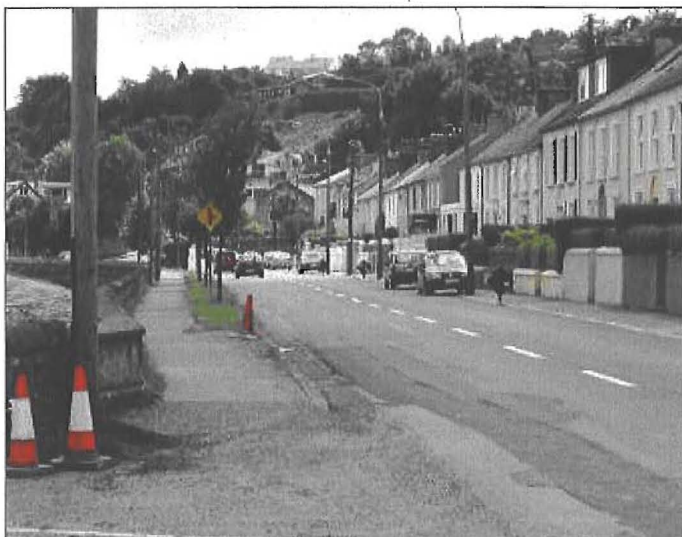
Plate A4 The R610 regional road linking Monkstown to Passage West. This is an area that would be affected by the proposed on-road pipeline network.
