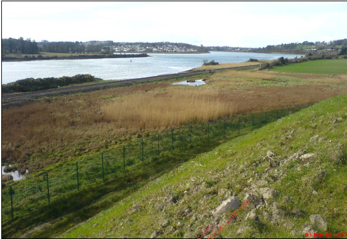
Plate 1 – Southern Edge of Construction Area on WWTP Site
