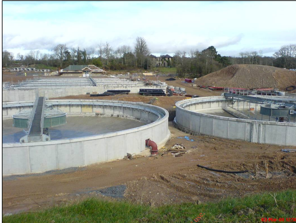
Photo 2: Looking north from southern edge of site to Springfield House.
