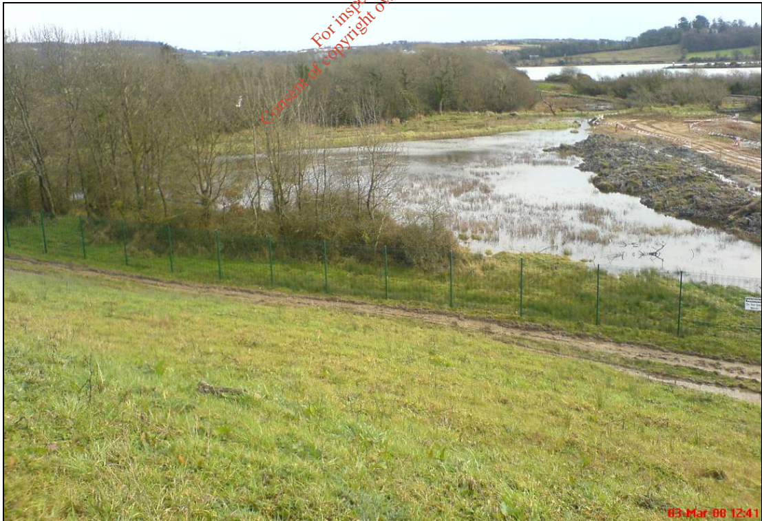
Plate 2 – Southwest Area of WWTP Site, showing Hardcore Road works
