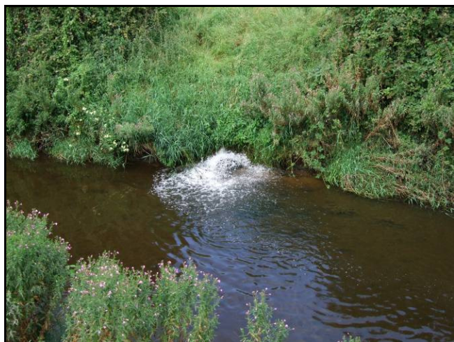
Plate 4 Primary outfall from the Mountmellick WwTP.
