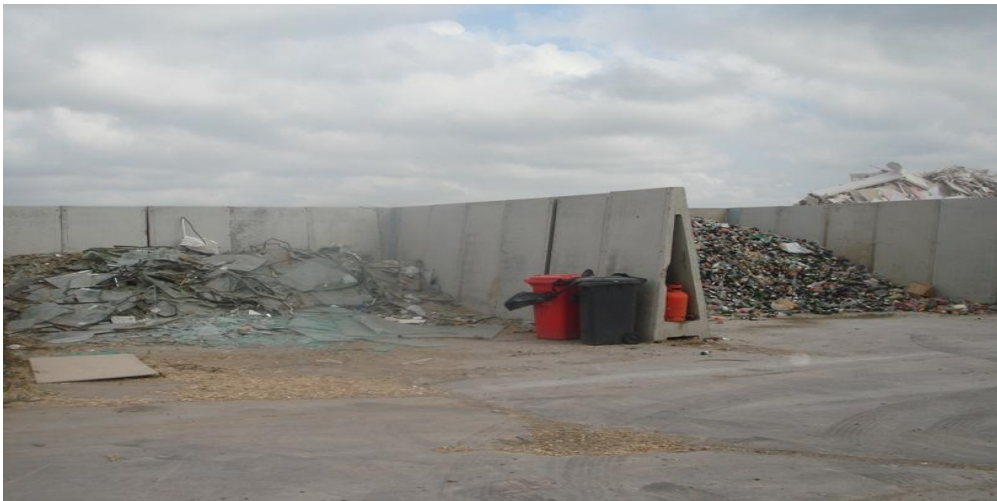
Image D.2: View of Glass Storage Bays
