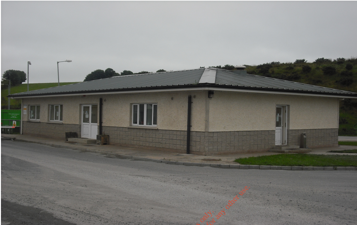
Figure 4 Administration Building at Corranure Landfill
