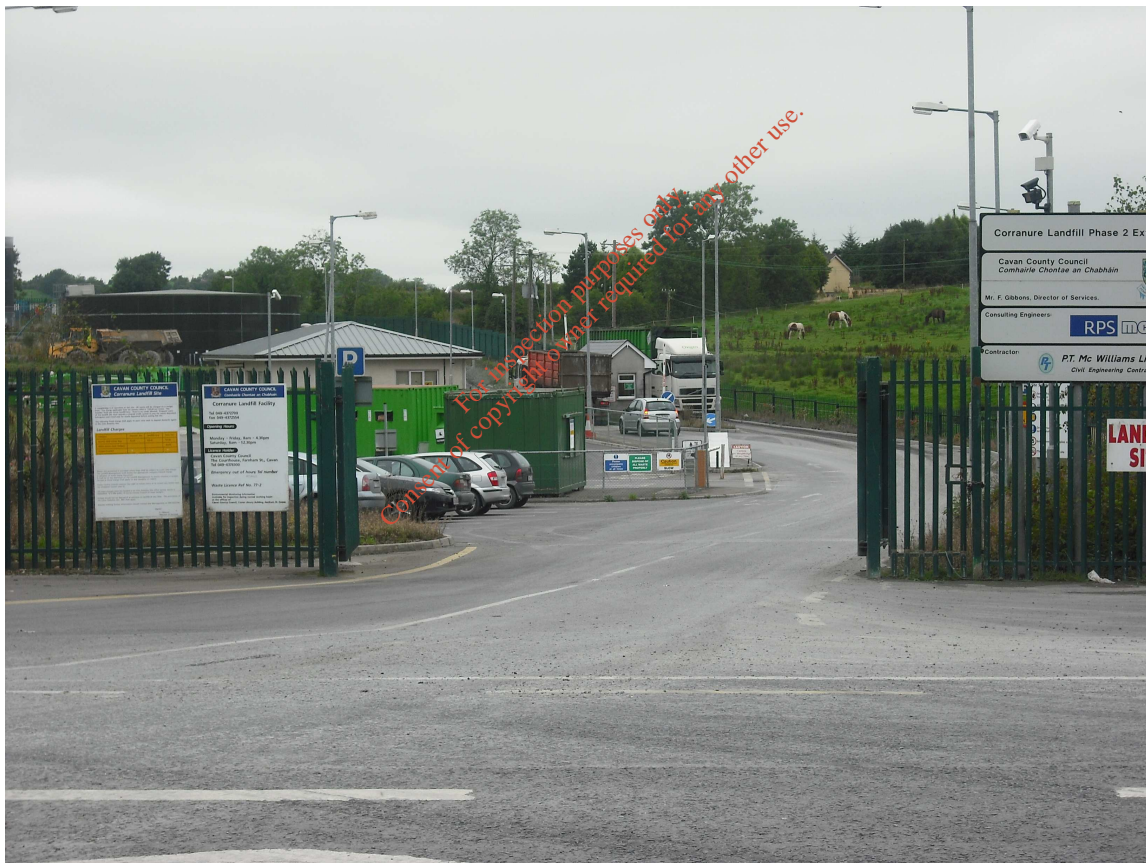
Figure 1 Entrance to Corranure Landfill
