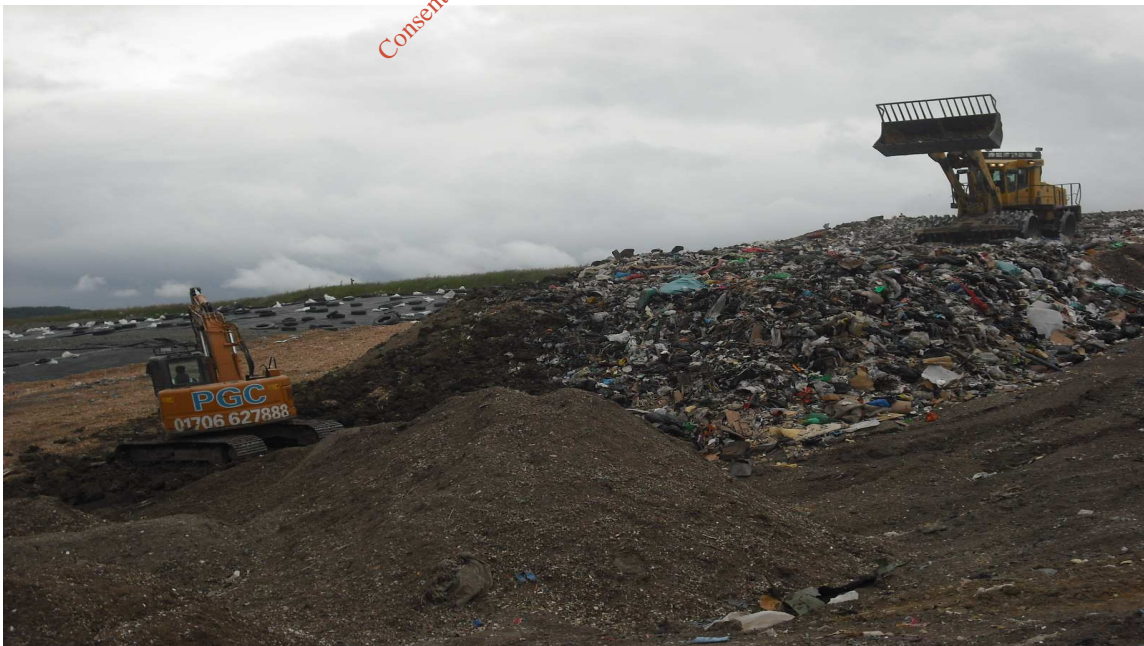
Figure 7 Landfilling of Waste Cell 3
