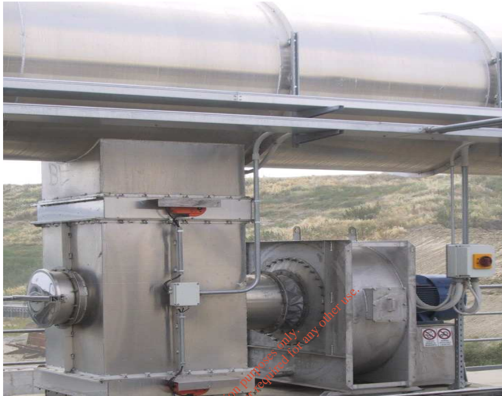
Figure 11 Typical Odour Control System
