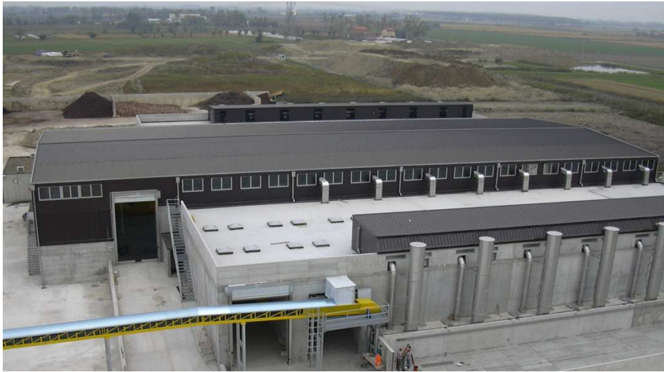
Figure 10 Typical Biological Treatment Facility
