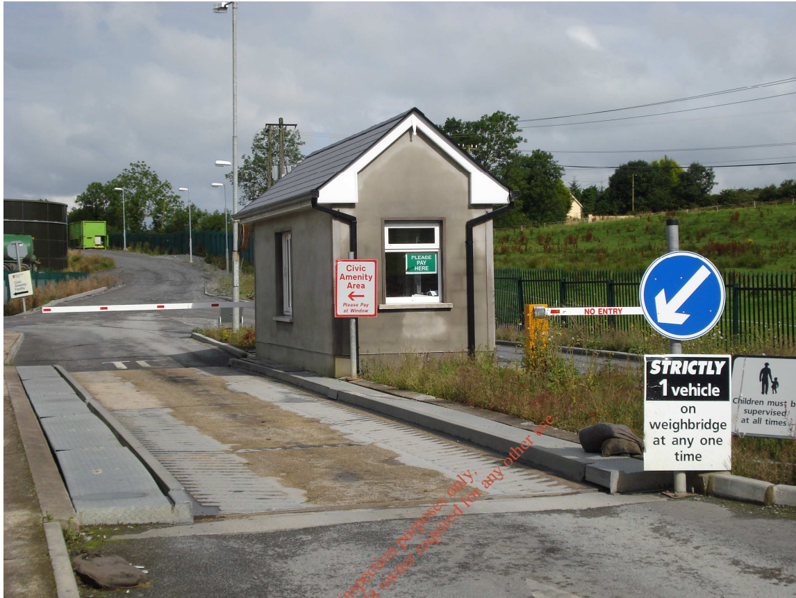
Figure 3 Weighbridge and Weighbridge Office
