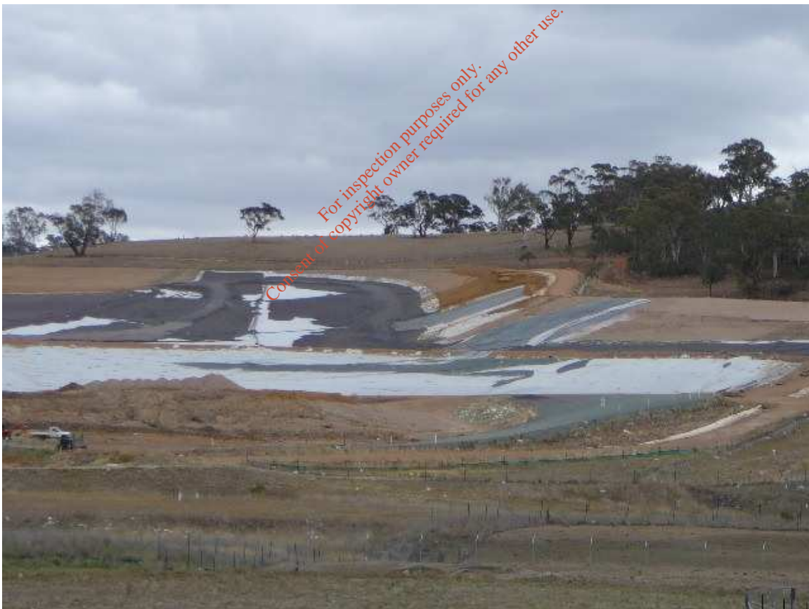
Figure 2.3.1 Typical Landfill Cell
