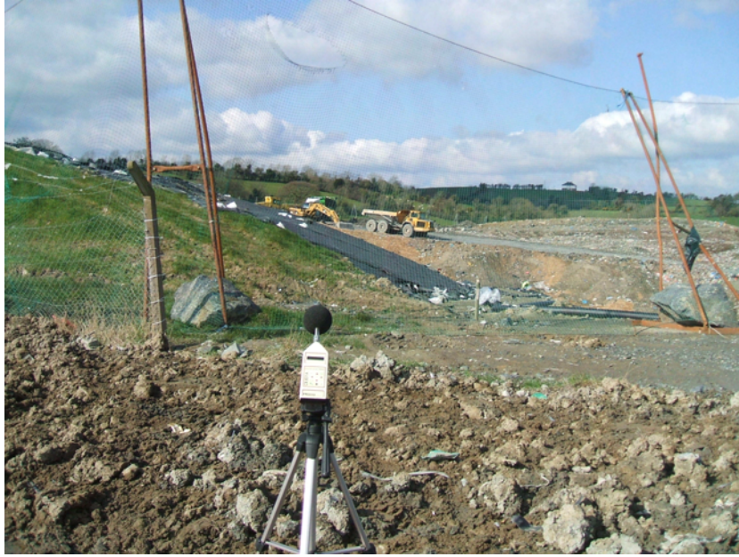
Noise monitoring equipment at B2
