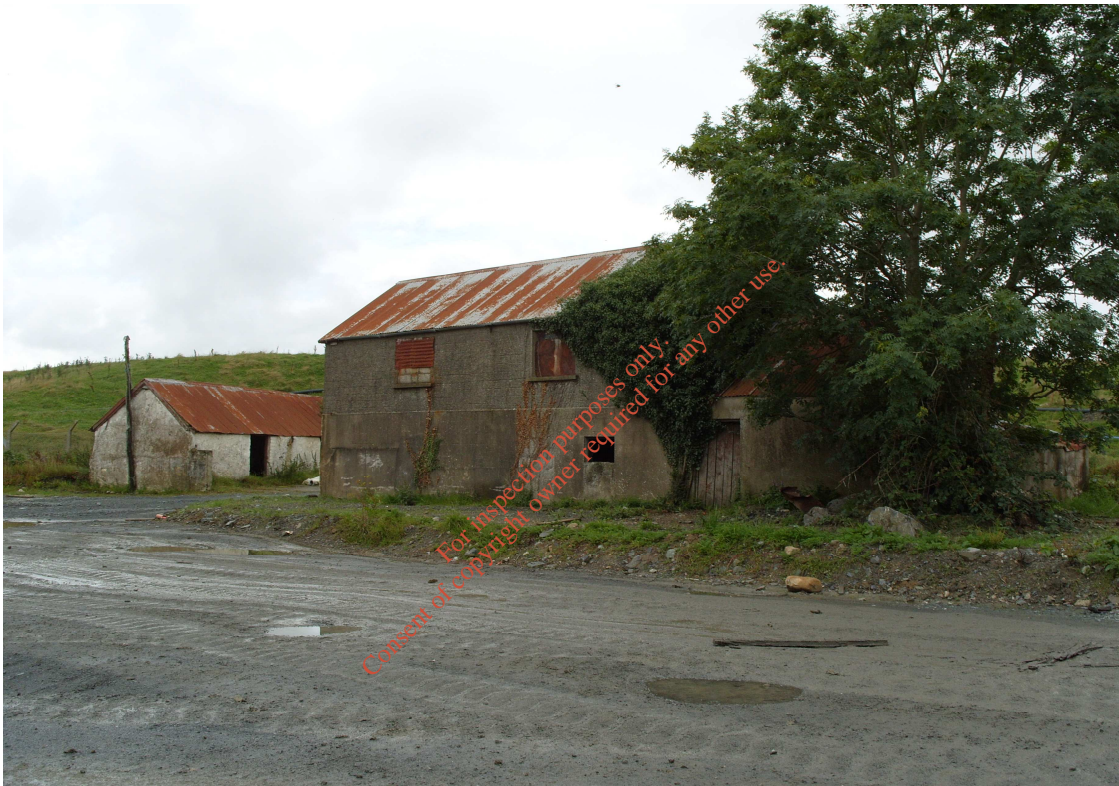
Figure 1 - abandoned house/shed occurs in the west centre of the site
