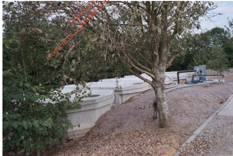
Photograph 3.6 Storage Tanks for Leachate from Landfill
