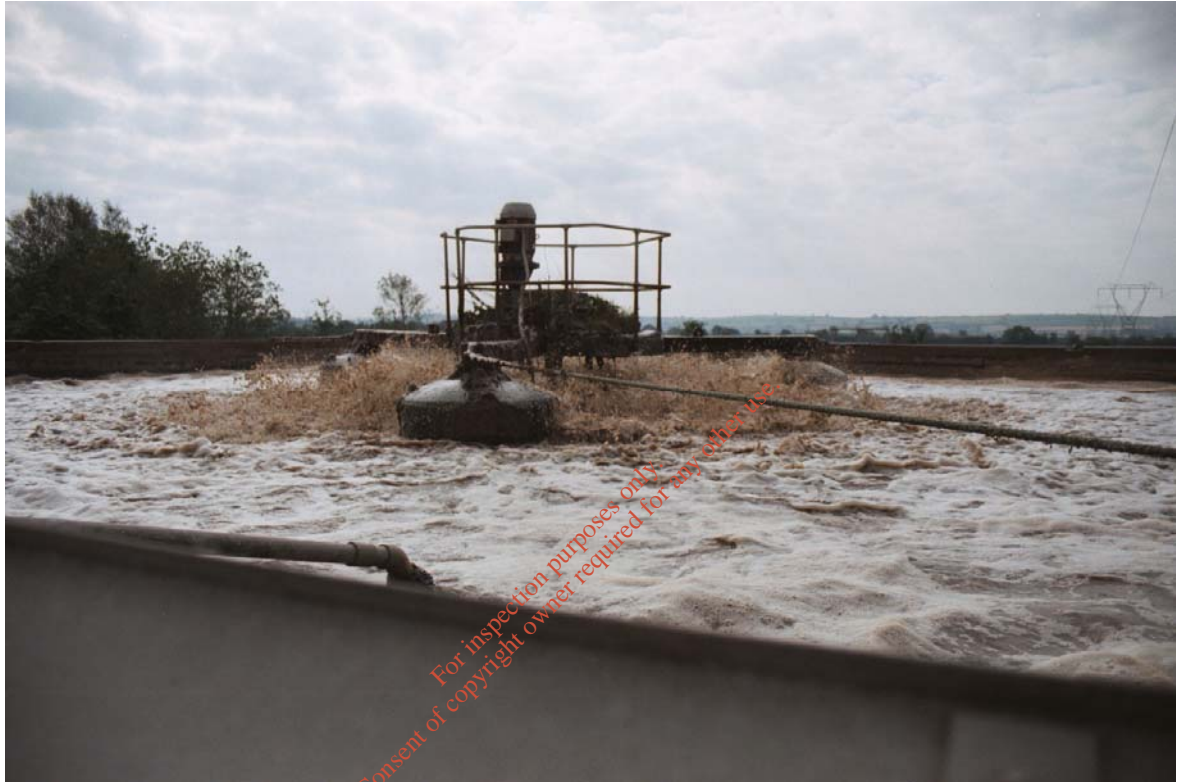
Photograph 1.2 Floating Surface aerator in Balancing Tank
