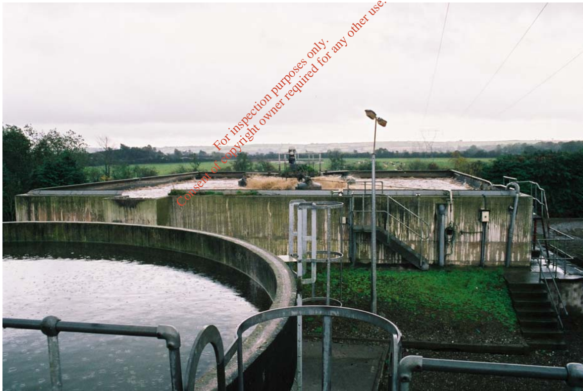
Photograph 1.1 – Balancing tank at the Carrigtohill works
