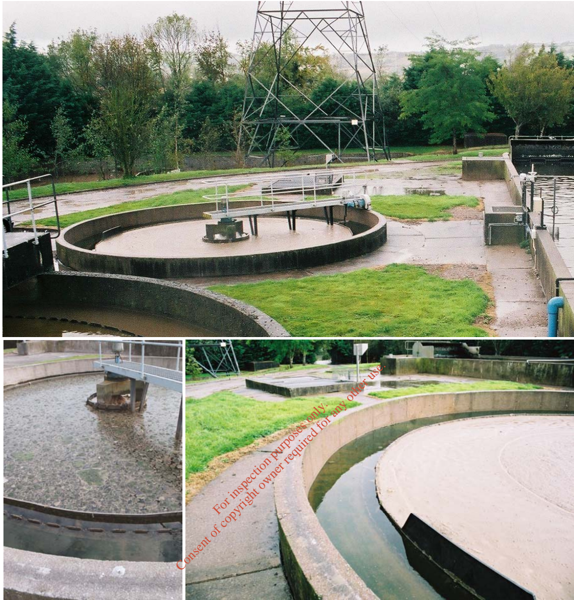
Photograph 3.4 Secondary Clarifier with Flow Measurement Chamber in Background
