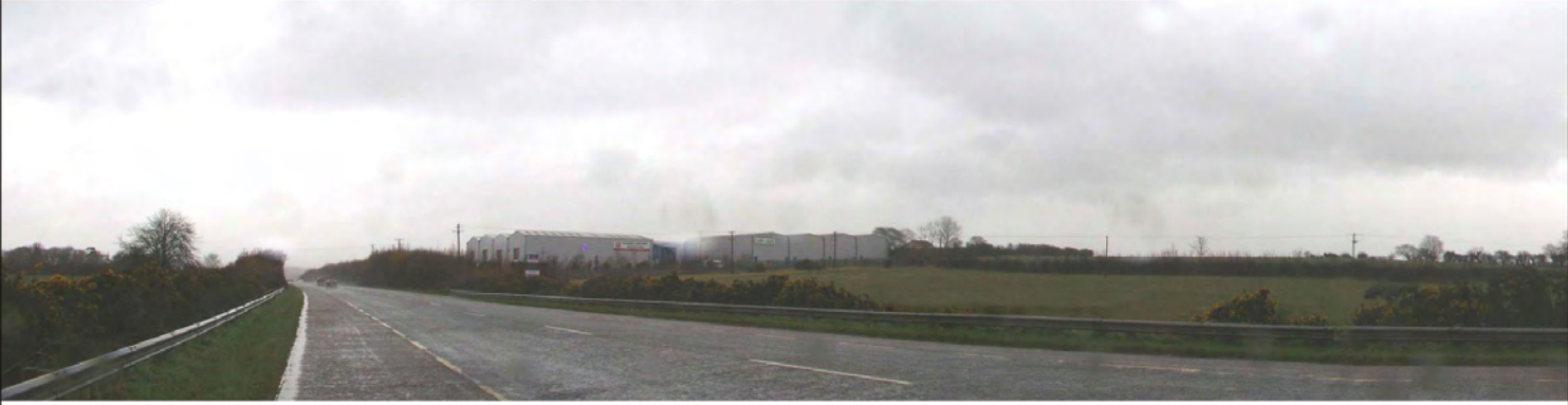
[VIEW-8] N11 LOOKING NORTH EAST, EXISTING PRIOR TO CONSTRUCTION
