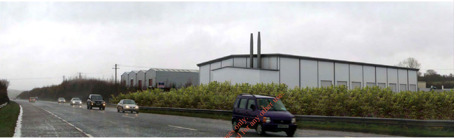
[VIEW-7] N11 LOOKING NORTH EAST, ARTIST'S IMPRESSION OF BUILDINGS, FIRST YEAR OF LANDSCAPE PLANTING
