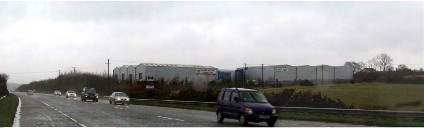
[VIEW-7] N11 LOOKING NORTH EAST, EXISTING PRIOR TO CONSTRUCTION
