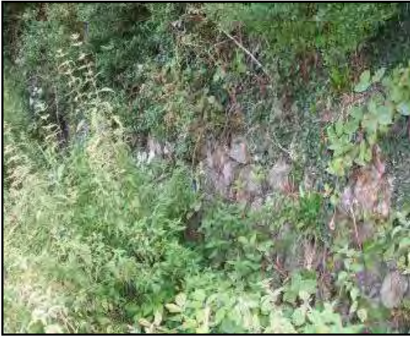
Plate 4 Stone wall located on the eastern boundary of the site
