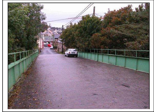
Plate 7. Iron bridge on Chappel St, from E
