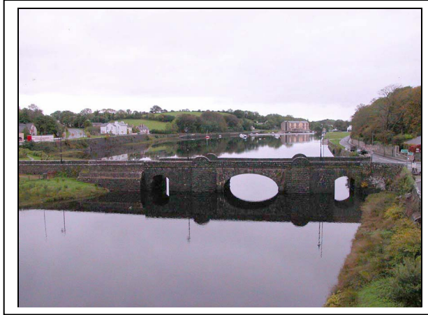
Plate 18. Viaduct, from E
