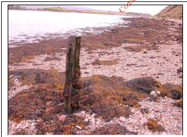
Plate 28. Modern timber (railway sleeper) Rosmore outfall, inter-tidal zone, from SE
