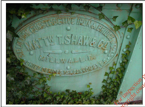
Plate 8. Detail on iron bridge, from S
