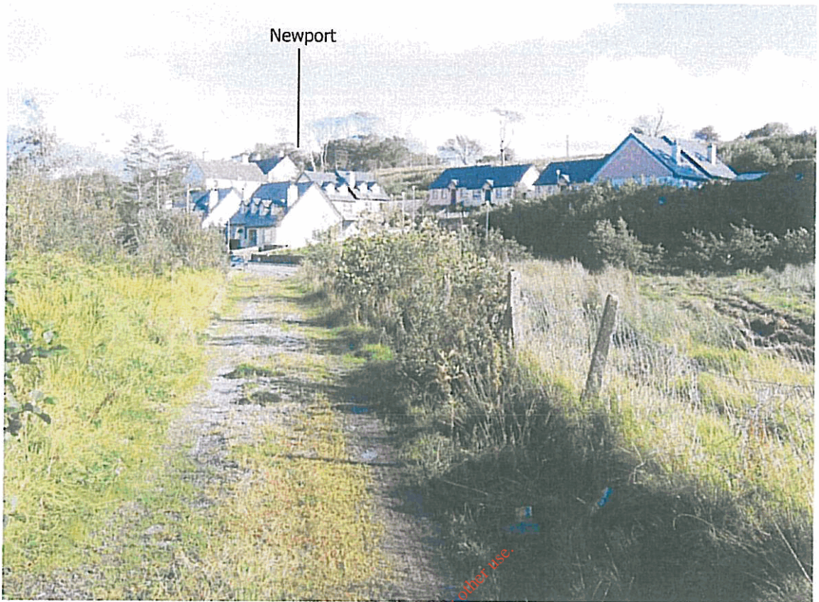
Photograph 3. An existing track extends from Newport town towards the Waste Water Treatment Plant site, overlooked by nearby houses. This will be widened and upgraded, forming the start of the proposed Access Road to the Waste Water Treatment Plant.
