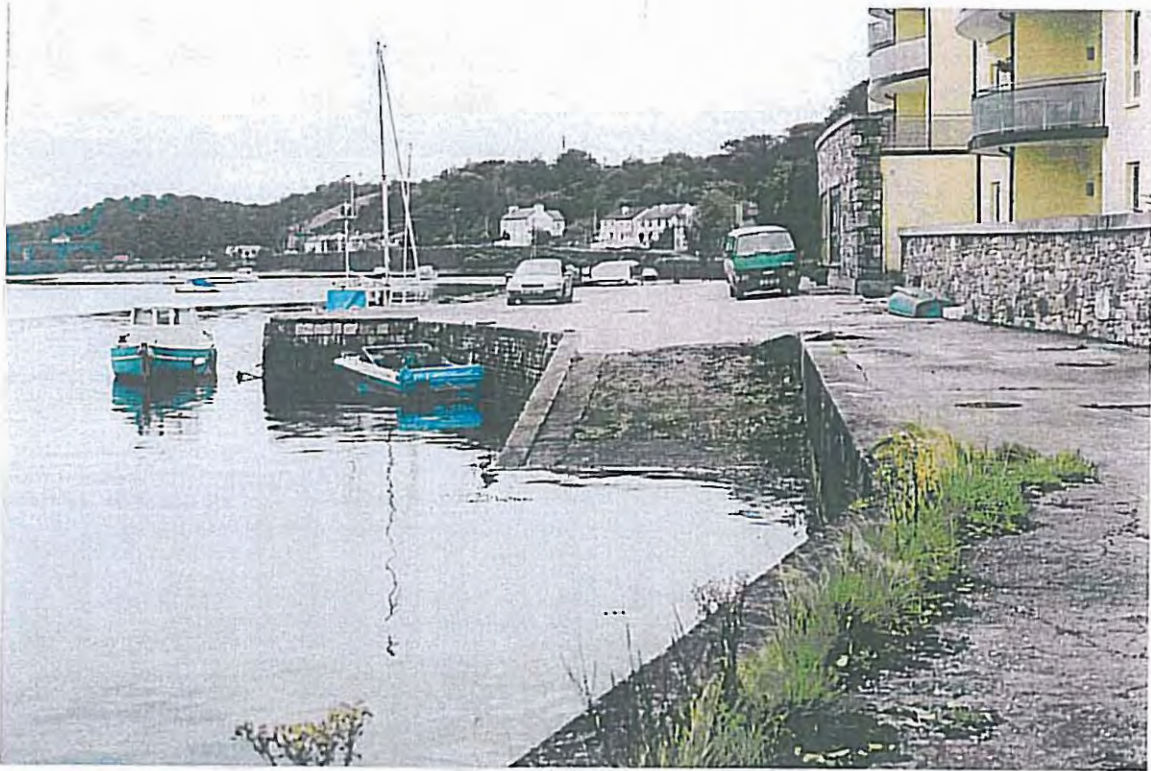
Plate 21. The pumping station linked to the rising main would be built on existing developed land associated with the harbour area and new apartment block.
