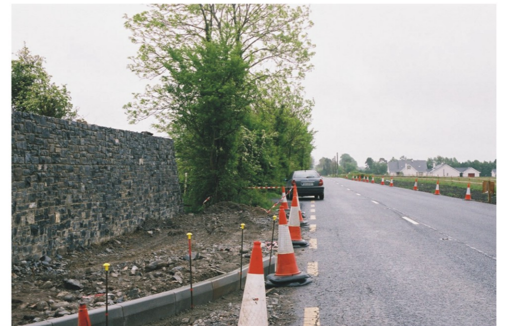
Plate 16: View southeast along the R403 from site entrance.
