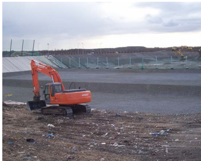
Landfill Cell at Drehid Waste Management Facility
