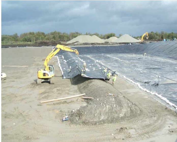
Overview of construction of landfill base
