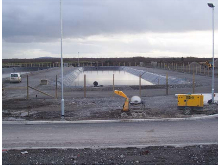
One of the Existing Surface Water Lagoons
