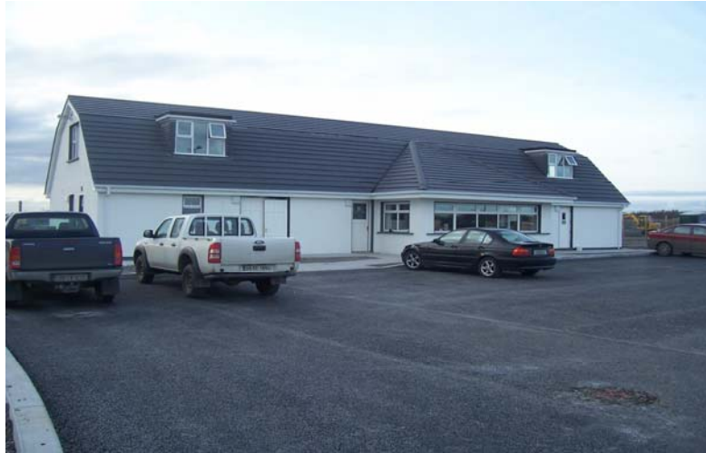
Administration Building at Drehid Waste Management Facility
