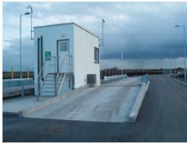
Existing Weighbridge at Drehid Waste Management Facility
