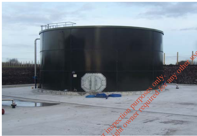
Leachate Holding Tank at Drehid Waste Management Facility
