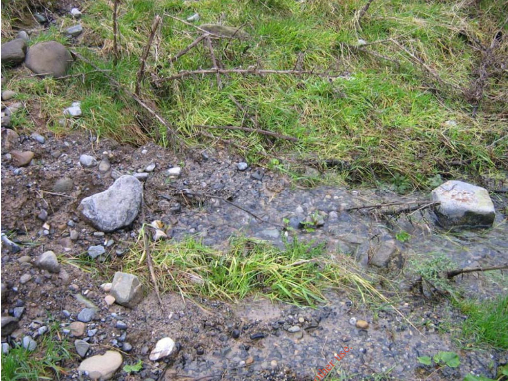
PLATE 6.3 Spring Emergence from Side of Existing Slope
