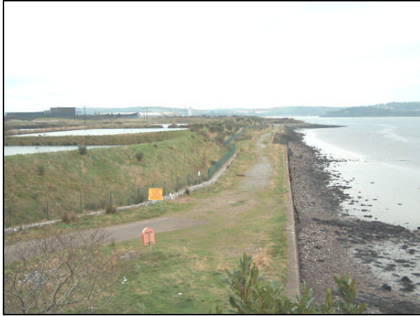
Plate 7: 'Right of way' at SW side of site, looking E from area of grotto / lodge.
