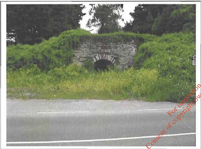
Plate 3.7. Pipe route flanked by CH5 along Monstown Creek road, from south
