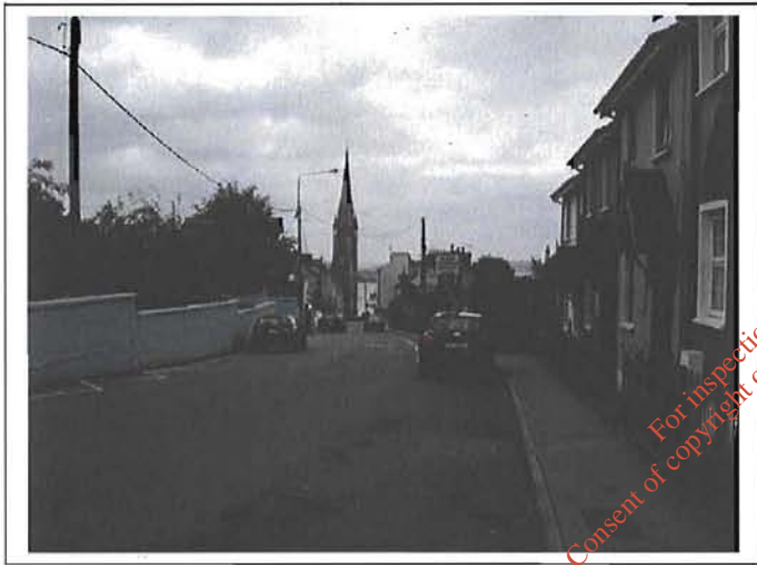
Plate 3.31. Pipeline route north of Cobh town centre, from north
