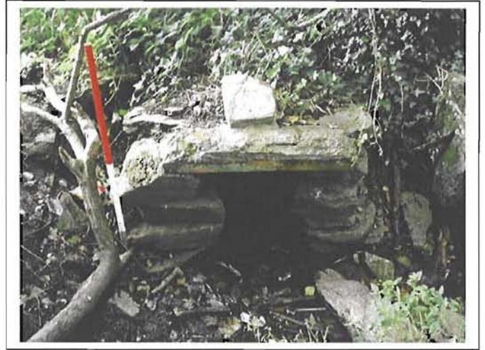
Plate 3.36. CH2, from east
