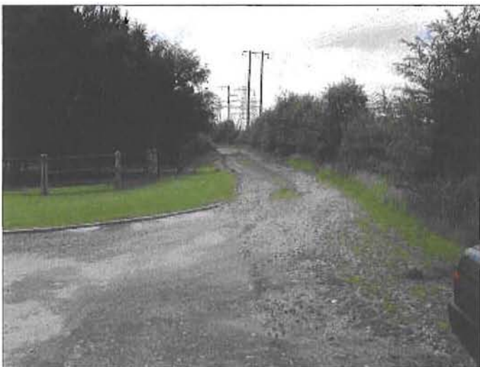
Plate A3 Artificial surfaces - the roadway leading into the proposed wastewater treatment plant site.
